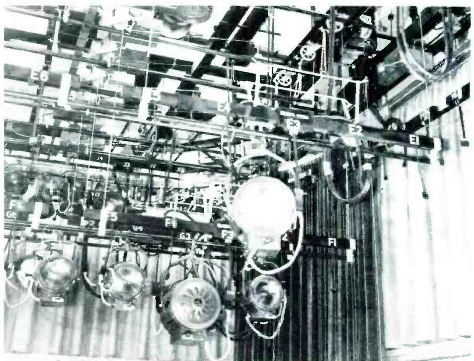
Figure 5. Adjustable batten suspension system.
