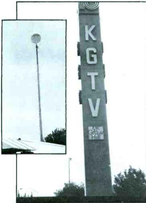
KGTV's new steerable Miniscan is installed at the station for ENG pickup.
