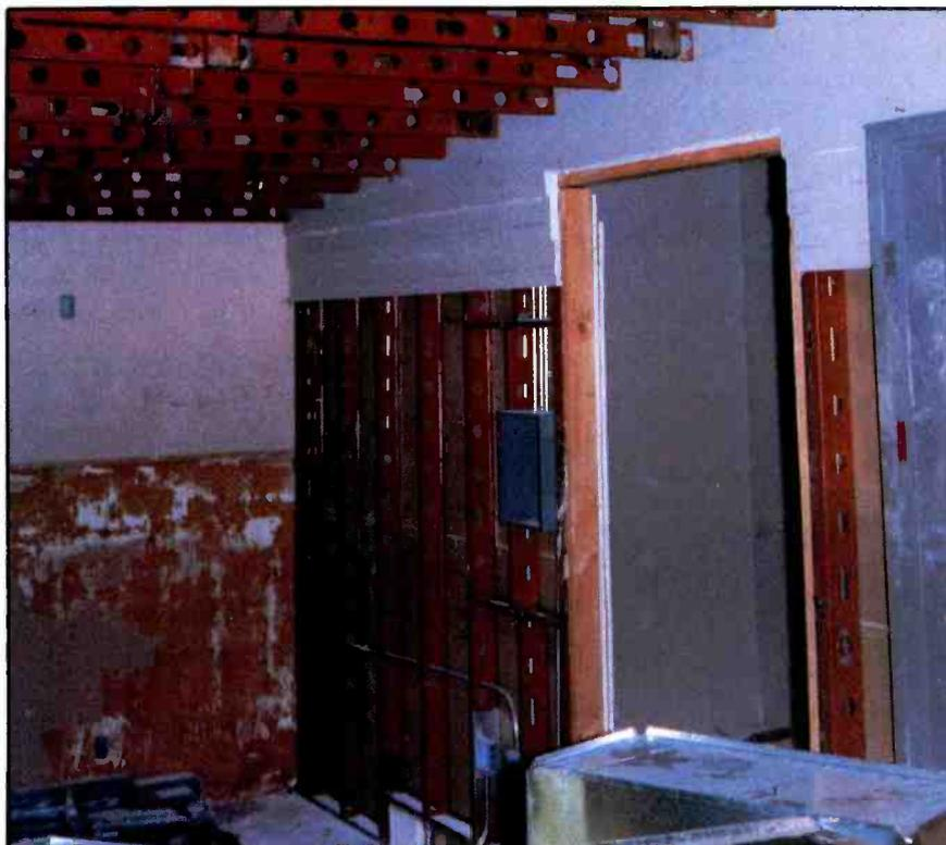
The Studio 4 audio mixing room under construction. Note the sloping ceiling and three layers of overlapping drywall. The studs are 14-gauge steel.
