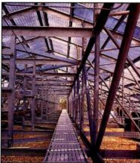
*An interior shot of the galvanized steel ice trusses.*
