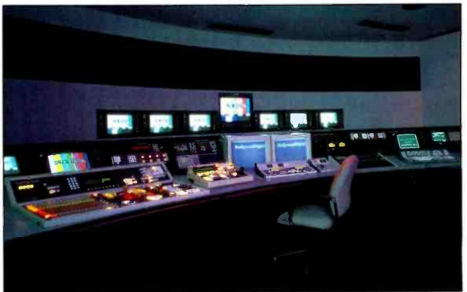
The curved wall behind the countertop provides proper acoustic backdrop for the speakers, which are hidden behind the black fabric just above the video monitor.
