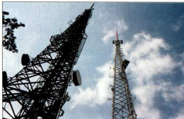
Sites with multiple antennas, and/or multiple towers will need to manage the total RF output, especially those sites with antennas located near ground level.
