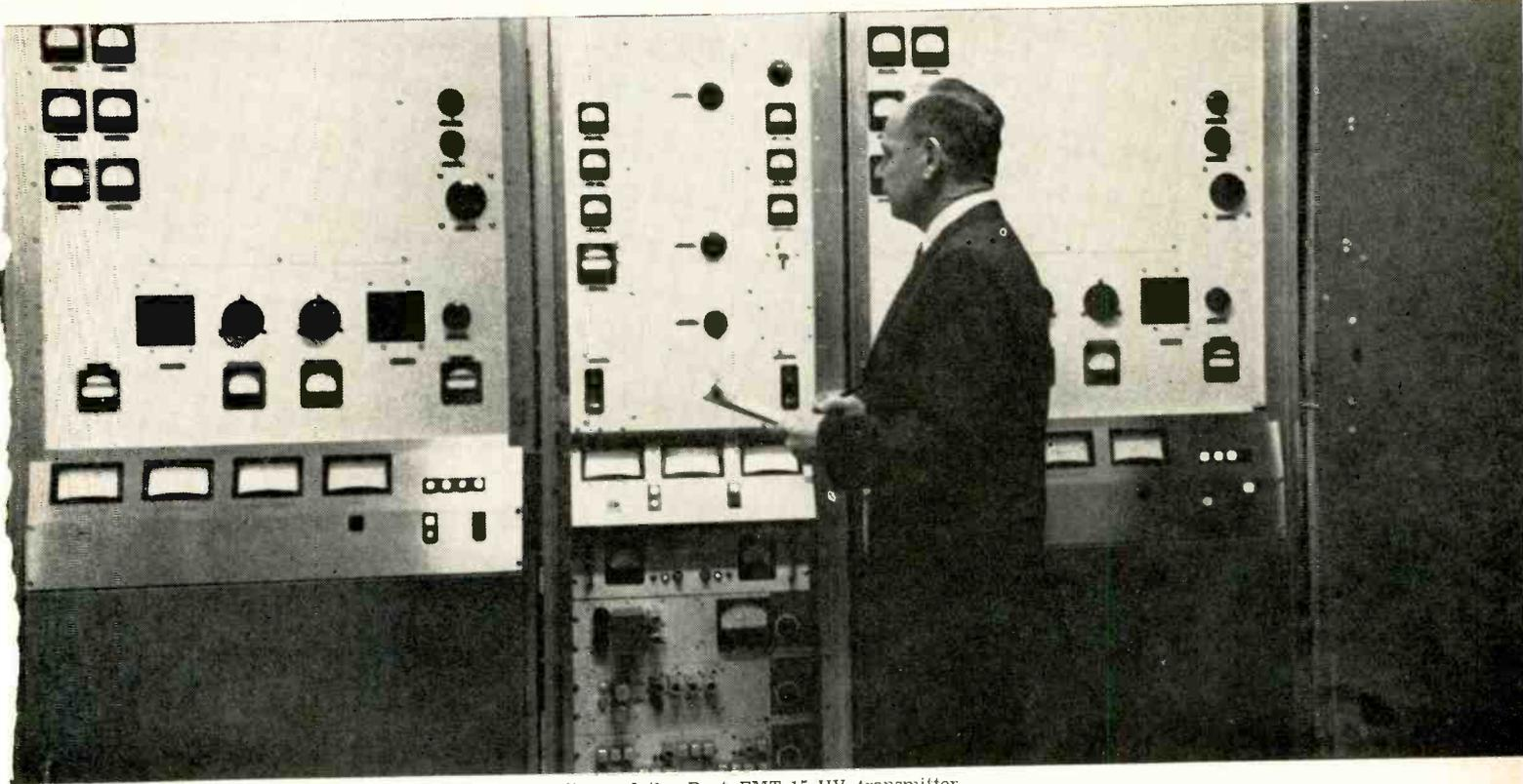
Chief Engineer Gordon Swan logs meter readings of the Rust FMT-15-HV transmitter. Twin 15-kw final amplifiers feed separate transmission lines.
