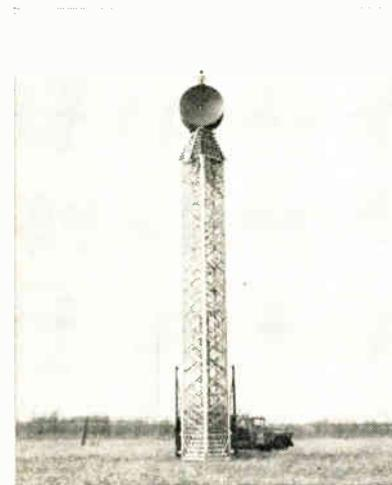
Stacked sections are pulled upright by tower guy wire. Rising sections pull remaining guys into place. No extra equipment required. No scaling of tower necessary. All erecting is controlled from ground level. Easily erected by five man crew.
