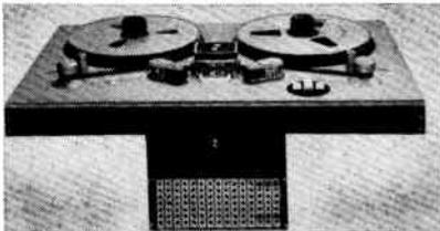
ideal anhysteretic magnetic recording process. A tight loop dual capstan drive system holds wow and flutter within 0.25% peak-to-peak from 0.1 to 10,000 Hz. Several configurations are available from 2 to 8 track ¼-in. and 0.150-in. (3.8mm) tapes. In rewind fast forward mode duplicator loads a 2400-ft NAB metal or plastic reel in 80's.
