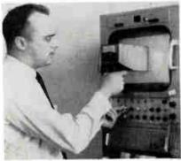
by a preset color temperature that allows broadcast engineers to adjust monitor controls for each color until the Colorgard meter indicates that the correct balance is being displayed on monitors.
