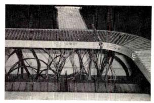
Inter connecting cable is carried in trays suspended from the first floor, as shown in this basement view, instead of more conventional floor trenches.
