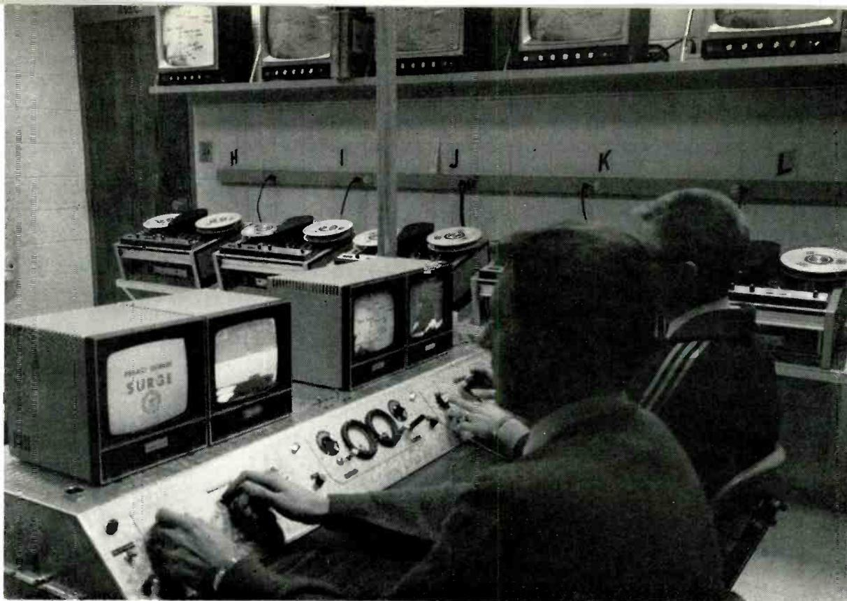
Operators monitor SURGE program that originates live in classroom for taping on 18 Ampex 5100 helical VTRs.
