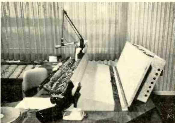
Entire wiring is accessible by hinging cart machines up and console panel down.
