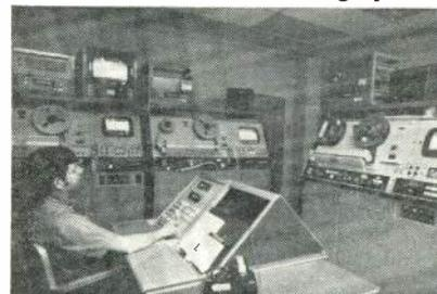
(shown above) along with three Ampex VR-2000 videotape recorders, all under control of a Jefferson Productions engineer.
