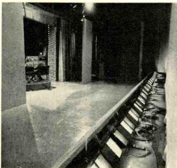
Fig. 2. Lights located below the cyclorama.
