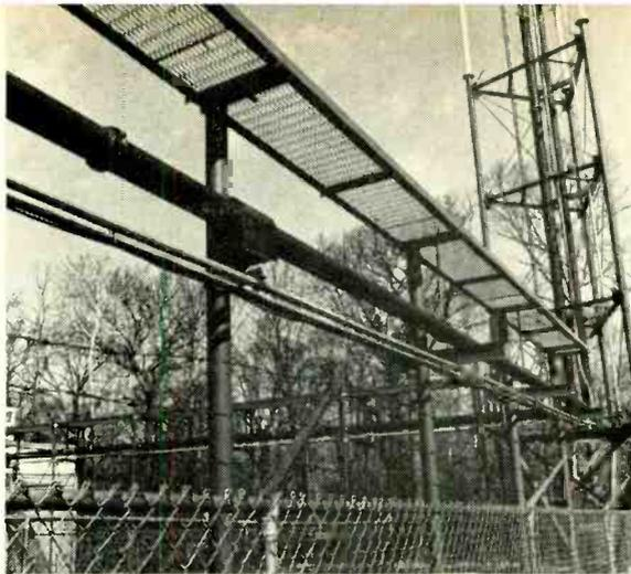
The HFE coaxial transmission line for a typical run of about 1000 feet is less expensive than dry-type or waveguides.
