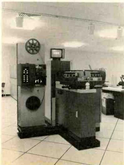
Fig. 8—Film island also in master control, includes a Cohu film camera, Eastman 16mm projector, Spindler and Sauppe slide projector. Film island includes a Super 8mm projector as well, for faculty who bring in material in that form.
