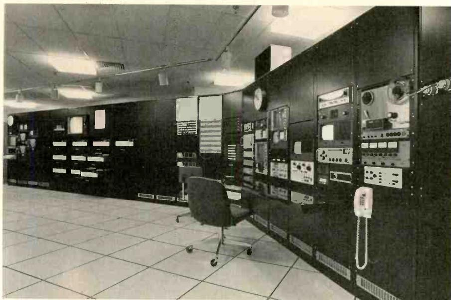
Fig. 7—Overall view of one wall of master control room shows, at far left, bank of U-Matic duplicators, patch panels in center, switching, control, monitoring in right wall. Room has 2700 square feet. Also facilities for VTR recording and post production.
