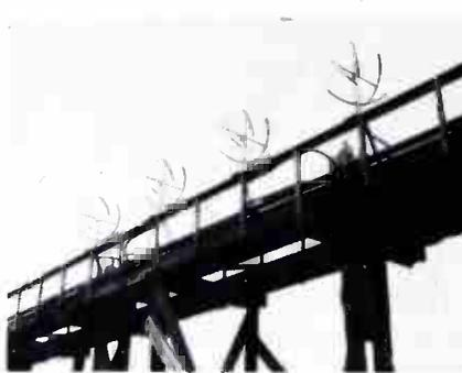
Rocamora, RCA antenna engineering manager, said that the new design is cheaper than a panel-type unit, has lower wind loading. The antenna will have eight bays, each with radiators more than twice as large as those in previous single-station antennas of the type. The photo shows several of the antenna bays under test at RCA's Gibbsboro antenna facility.
