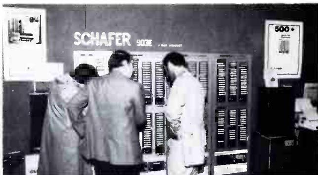
(Above) Schafer 903E full-automation system, introduced at NAB in Chicago, has extended memory for three full days of automatic programming. System shown has six Audiophiles, each holding 48 carts all available for automatic play.
