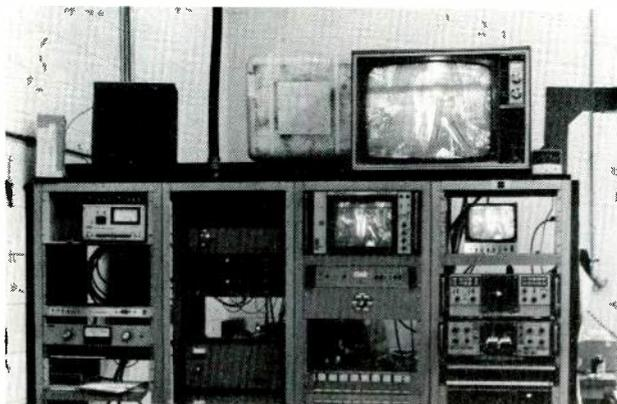
Monitoring, processing and test units are installed in rack adjoining the transmitter.
