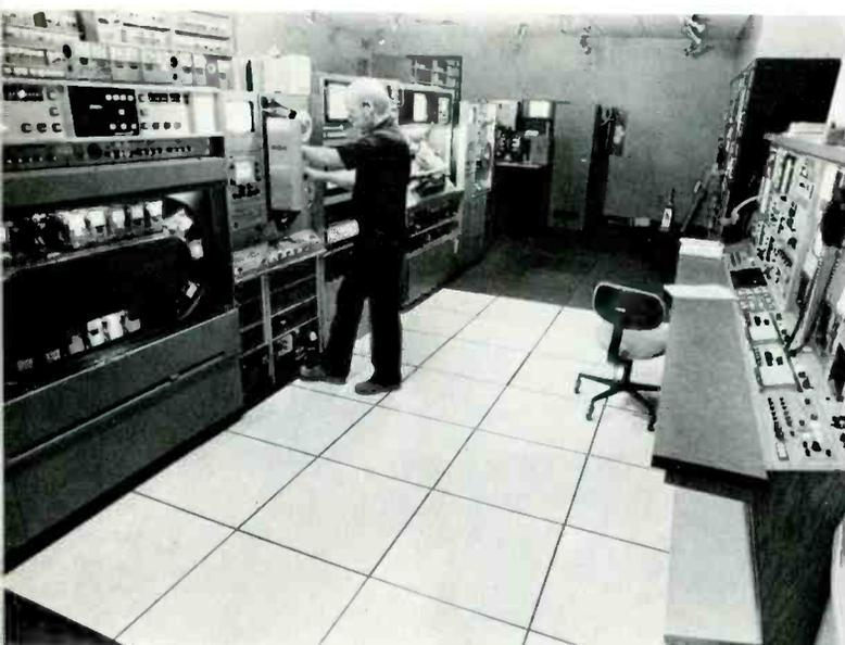
*Machine room is spacious and efficient. Computer flooring is used for ease of access to wiring.*
