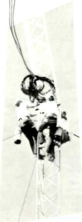
Far surpassing steel guys in strength and durability, PHILLYSTRAN is manufactured from impregnated KEVLAR\* and polyurethane. Completely non-metallic, PHILLYSTRAN eliminates electrical problems and the usual problems of RFI.
