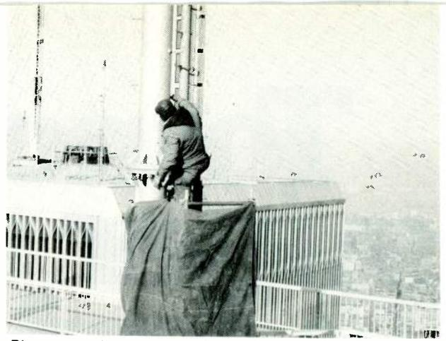
Rigger completes work on Bogner four-bay slot-and-dipole CP antenna for WTVG's 1000 W translator in south tower of World Trade Center, 1,398 feet above sea level. Note in background the north tower mast which will house an array of VHF antennas for the New York area
