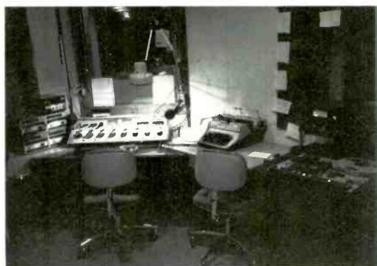
*KAAM's news control room. Each module serves two working newsmen with full cart and reel-to-reel recording of mic and telephone inputs*
