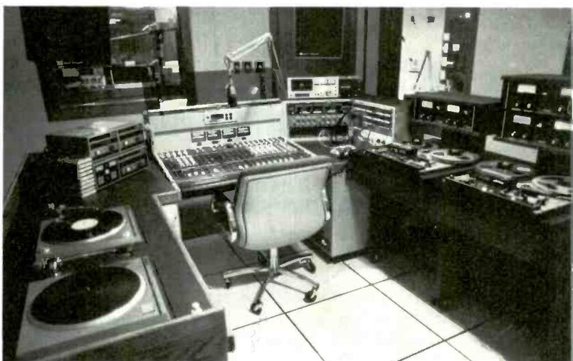
*KAAM's production studio. The facility features an Audionics Model 110A mixer, an Orban Parasound parametric equalizer, and an Eventide Clockworks harmonizer*
