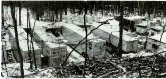
Whiteface Mountain was the venue for alpine skiing events, coordinated through a complex of mobile vans parked 1000 feet uphill from base lodge in a small clearing. Cameras on small wooden pallets could be transported from one slope to another by helicopter. For longer cable runs, special RF repeaters developed by Philips for its LDK cameras, used extensively at the venue, provided triax runs up to 15,000 feet
