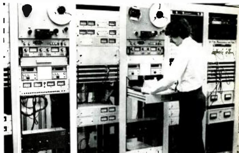
Chief engineer David Pollard makes adjustment in terminal room of new RKO network plant. Racks hold audio processing and amplifying equipment, cart and reel players, patch panels. Room can go on air if needed
