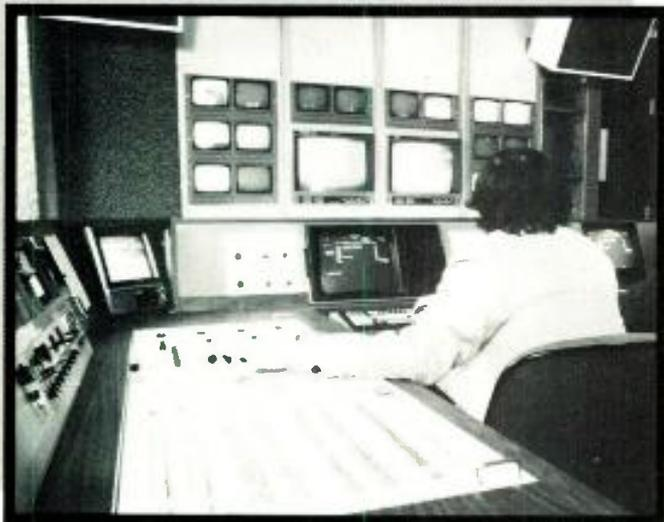
In ABC's new post-production room monitors are in wall above edit position, switching directly under operator's left hand.
