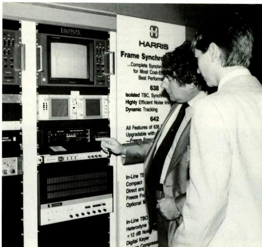
The new Harris model 642f frame synchronizer/time base corrector features up to 12 dB of Smart Noise Reduction that is automatically applied to the amount of noise measured in the video.
