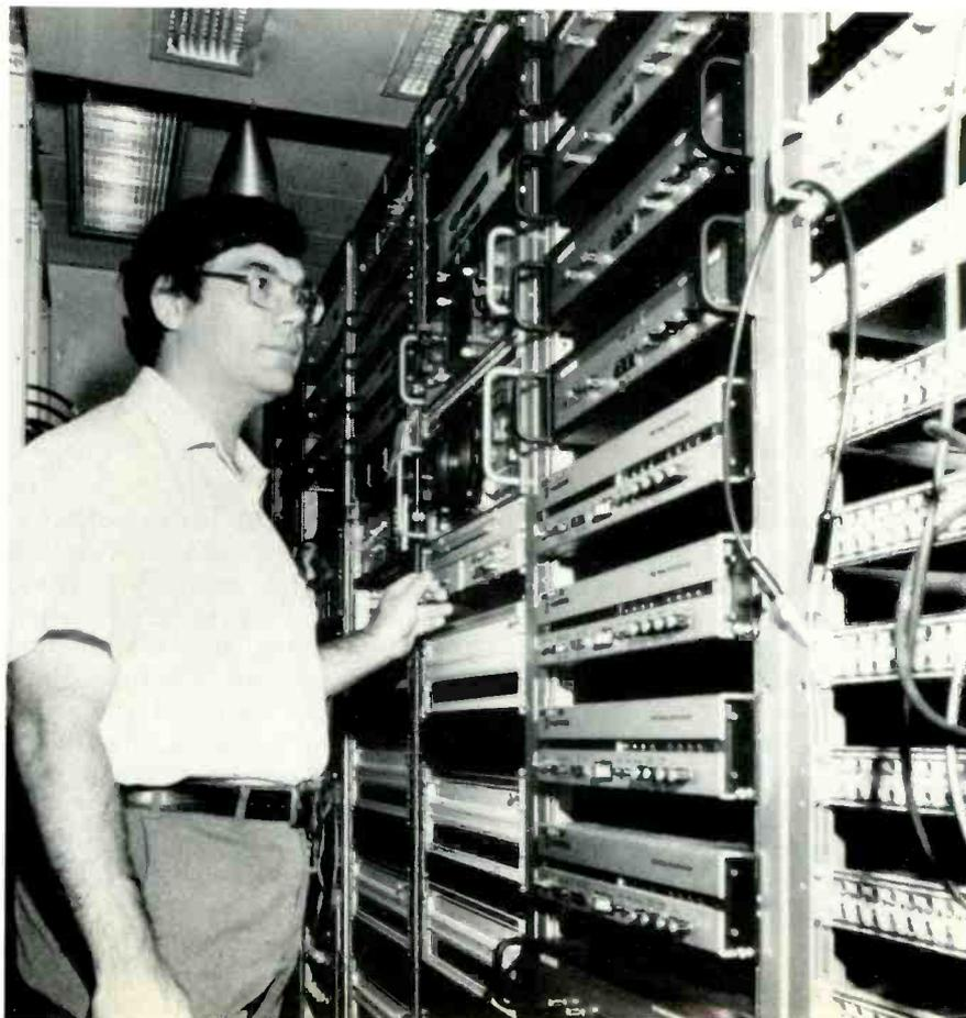
Outside video sources at WBNS-TV are synched soon after they enter the building. Dan Black, maintenance technician, surveys the station's Microtime and Harris frame synchronizers.
