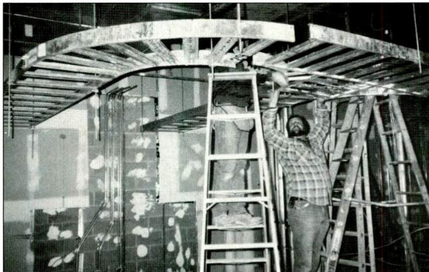
*Construction workers install video-signal and electrical conduits in the new ATTC laboratory.*
