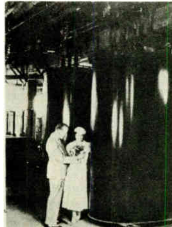
Modulation transformers weighing 37,000 pounds each were installed in the basement of the transmitter building. Circa 1934.
