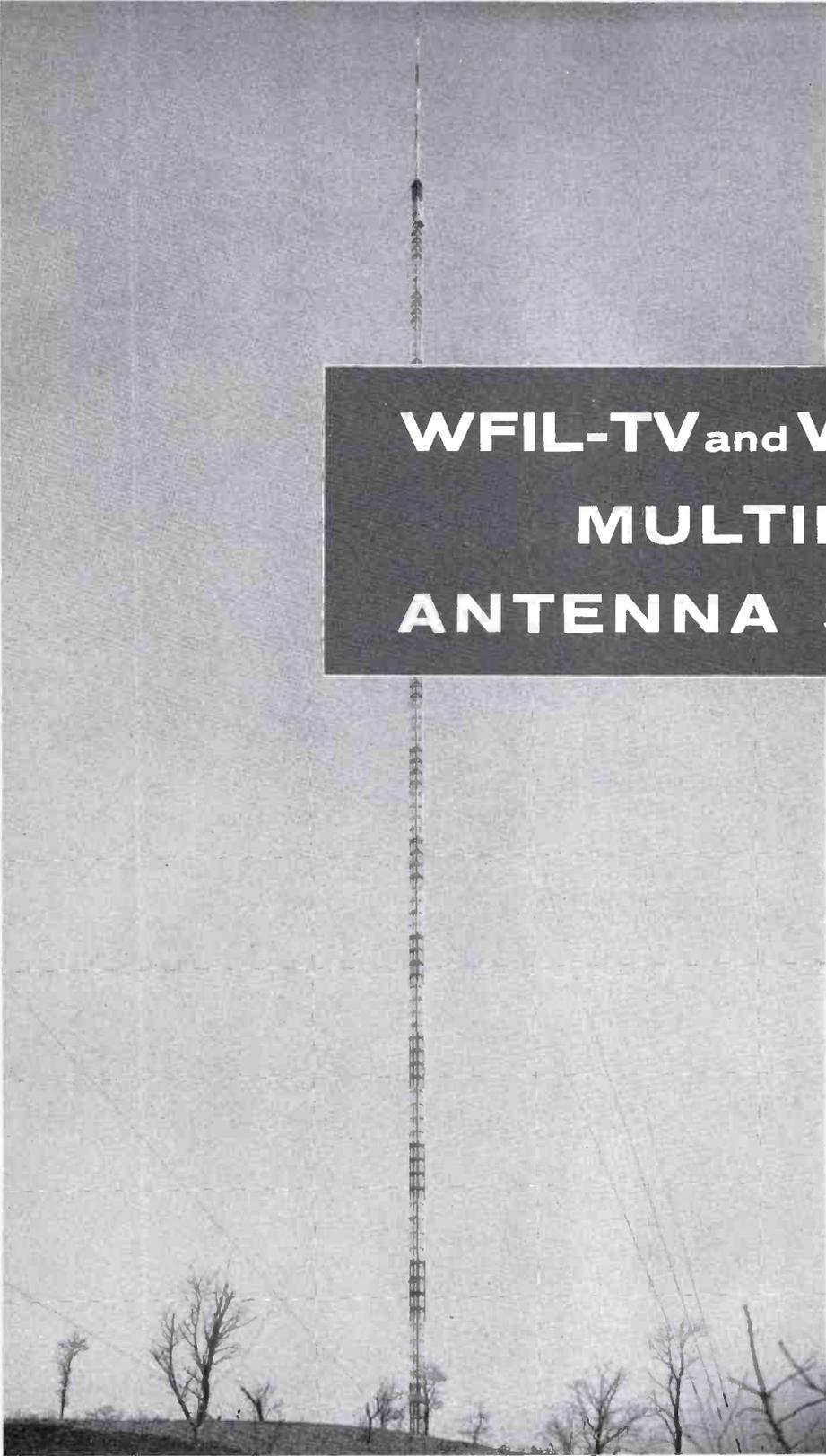
FIG. 1. Over-all view of the new WFIL-WRCV joint tower. The structure is 917 feet high, and the antennas increase the total height to 1109 feet.
