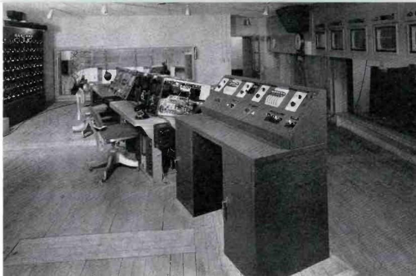
FIG. 12. The WTPA control room includes portable control units for three field cameras and controls, and two film cameras. Also housed here are lighting controls for both studios.
