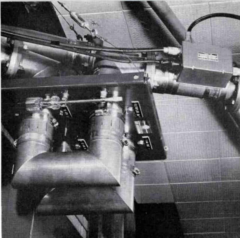
FIG. 3. Manual coaxial switching panel permitted rapid manual switching between 1 and 12 kilowatt outputs during conversion, and ultimately between 1 and 25 kilowatt outputs after conversion was completed.
