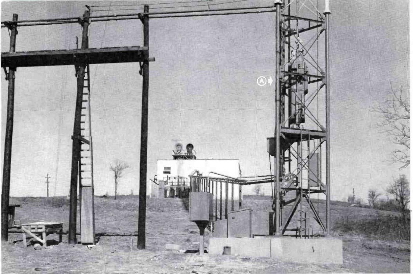
FIG. 4. Base of tower is an 11-foot deep, reinforced concrete foundation, six feet square with only two feet extending above ground. The two-man, radio-controlled elevator, noted by letter A, is shown in above photo.
