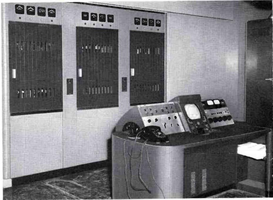
FIG. 7. Initial 1-kilowatt transmitter installation. A false wall provided room for expansion.
