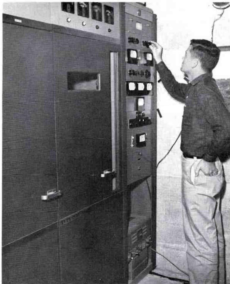
FIG. 16. View inside transmitter building showing engineer tuning speech rack (No. 3 rack). Cabinet No. 1 (extreme left) contains phasing equipment. Cabinet No. 2 is the BTA-500MX.
