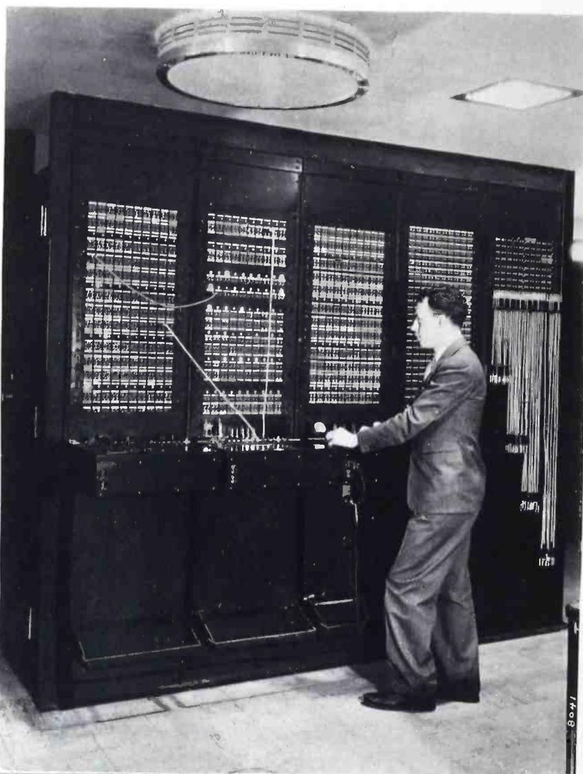
(ABOVE) LINE TERMINATING RACKS LOCATED IN THE MASTER CONTROL ROOM
