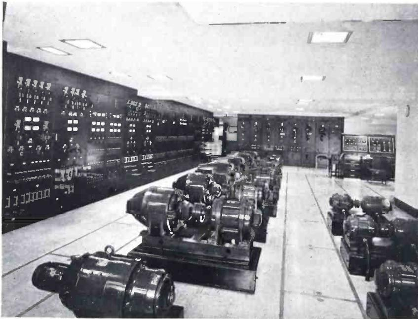
VIEW OF POWER ROOM SHOWING THE TEN MOTOR GENERATOR UNITS, SWITCH-BOARDS AND POWER CONTROL DESK
