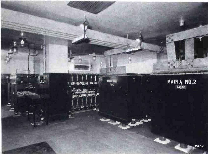
"FIFTY TONS OF STORAGE BATTERIES." THE HEAVY METAL BARS CARRIED ON THE CEILING INSULATORS ARE THE 14-VOLT BUSES
