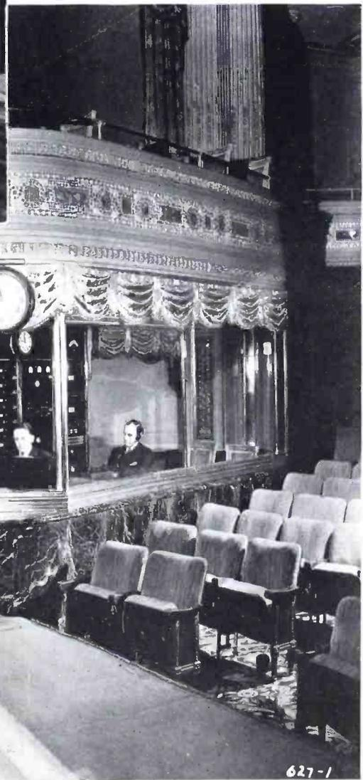
CONTROL ROOM OF COLUMBIA RADIO PLAYHOUSE, BUILT INTO THE ORCHESTRA BOX SECTION AND BEHIND DOUBLE-GLASS PANELS. THE EQUIPMENT RACKS ARE SEEN IN THE BACKGROUND, THE MIXER CONSOLE IN THE FOREGROUND. RCA VICTOR STUDIO EQUIPMENT INSTALLED THROUGHOUT
