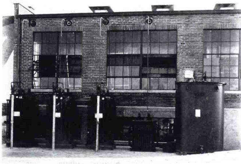
THIS VIEW SHOWS THE MAIN PLATE TRANSFORMERS, FILTER REACTOR, AND MODULATION TRANSFORMER
