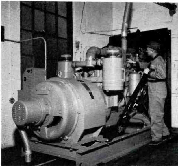
FIG. 11. WRVA 50-kw dummy antenna with covers removed, showing a special matching network on the left with the water-cooled dummy load on the right. This equipment was specifically designed by RCA for WRVA.
