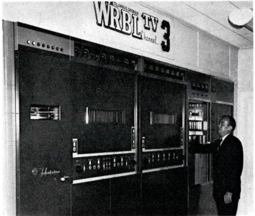
FIG. 8. WRBL-TV employs 25-kw Type TT-25CL TV transmitter.
