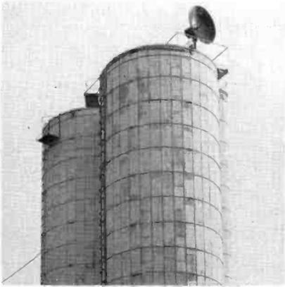
FIG. 10. Microwave antenna is mounted on silo at farm for link with TV studio.
