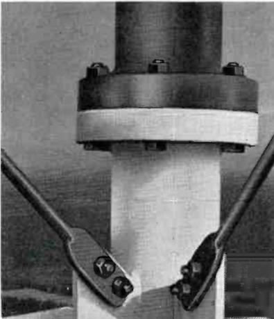
FIG. 11. Side-mounting of temporary channel-9 antenna.
