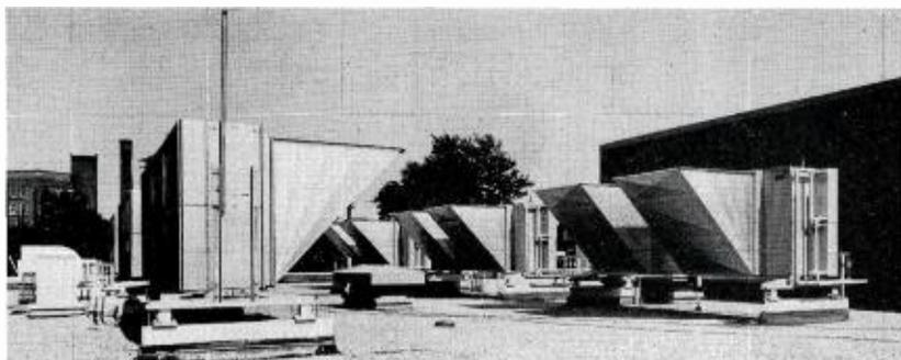
**FIG. 30.** Each compressor has its individual air-cooled condenser on the roof. No cooling tower is used. Each condenser has two 48-inch fans, belt-driven by one 3 h.p. motor. This system eliminates the problems of corrosion, algae control, water and sewer-tax costs, freeze-up protection.
