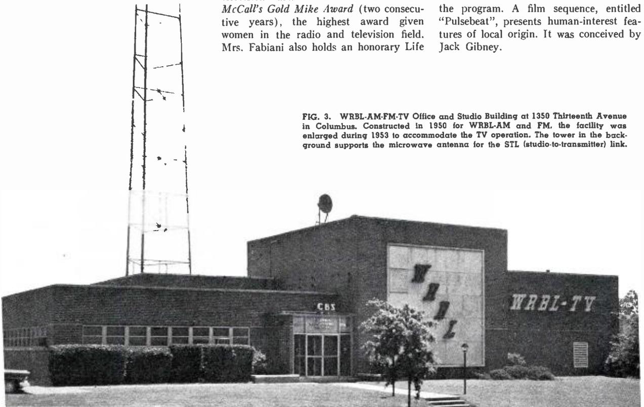
FIG. 3. WRBL-AM-FM-TV Office and Studio Building at 1350 Thirteenth Avenue in Columbus. Constructed in 1950 for WRBL-AM and FM, the facility was enlarged during 1953 to accommodate the TV operation. The tower in the background supports the microwave antenna for the STL (studio-to-transmitter) link.
