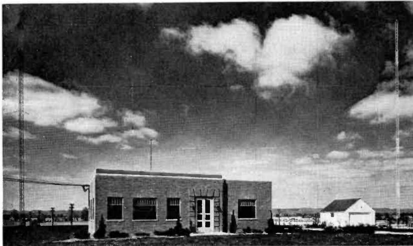
▲ FIG. 31. AM radio transmitter building in Jeffersonville, Ind. Note 2-tower array, at right and left. For normal operation, transmitter is remotely controlled from downtown Louisville studio.
