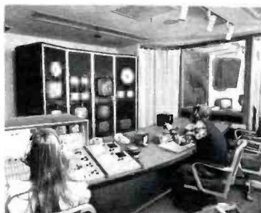
Studio A control facilities include 20-input audio mixer, and triple re-entry video switcher with dual effects and dual Chromakey.
