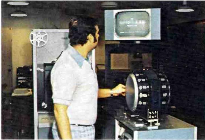
TK-28 film system permits integrating film and slides into tape productions without sacrificing quality.
