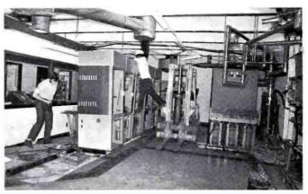
The veteran TT-50AH transmitter was disconnected and readied for removal.  $% \label{eq:controller}$
