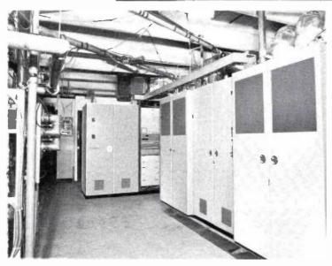
Ample room is provided behind cabinets for maintenance accessibility. Filterplexer and OPTO-Switcher are at left.
