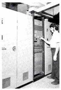
Remote control and monitoring rack is flanked by the two Power Supply cabinets. At WALA-TV, these are positioned at right angles to the front line cabinets.
