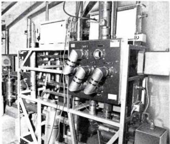
A new filterplexer (top) was installed with the TT-50FH, along with an OPTO-Switcher (bottom) which provides for easier and more versatile switching. The switching system is factory optimized for best VSWR.
