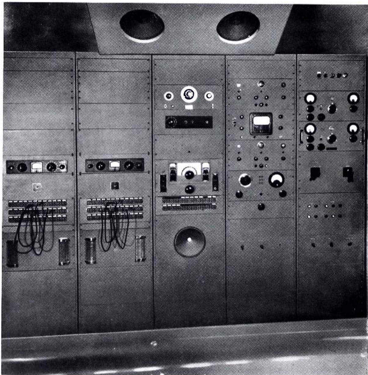
**FIG. 9.** Audio and measuring equipment cabinet racks employed at shortwave station WOOC and WOOW. Five racks are shown. Three of these house the audio and the monitoring equipment, and the remaining two are used to mount various measuring equipment and control panels.
