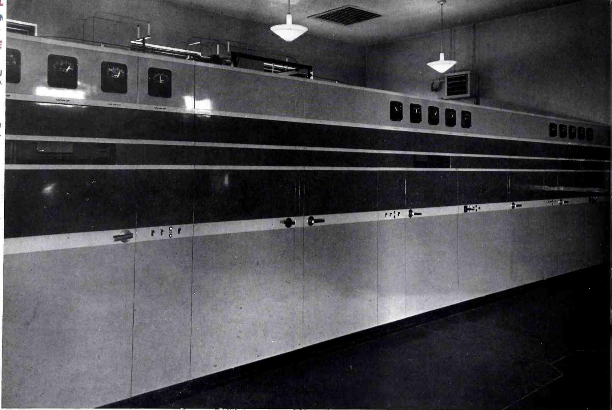
**FIG. 3.** *View of WOOC and WOOW transmitter panels at Wayne for the three RCA r-f channels; each channel consists of a complete exciter unit, from crystal oscillator to driver stage, including a 50 KW r-f power amplifier.*
