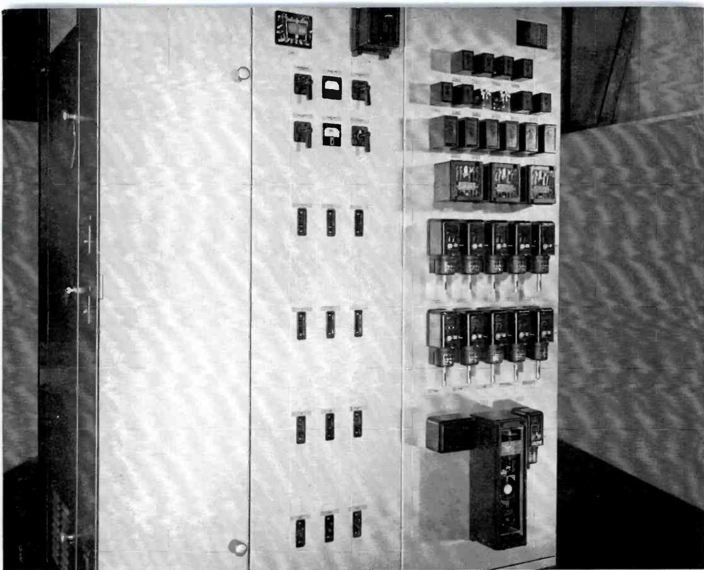
**FIG. 11.** All time delay relays, overload relays and distribution circuit controls are mounted on the control and distribution unit which is located just inside the righthand door of the transmitter. This is a totally inclosed unit which is designed, manufactured, and assembled according to best switchgear practice. The BTA-50F includes more advanced and more complete protective and control circuits than any transmitter designed to date.
