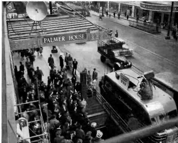
FIG. 10. Another camera, mounted on RCA Mobile Unit, was used to pick up crowds at hotel entrance. Note relay transmitter on marquee. It was used to send convention pickups to WBKB for on-air telecasts.
