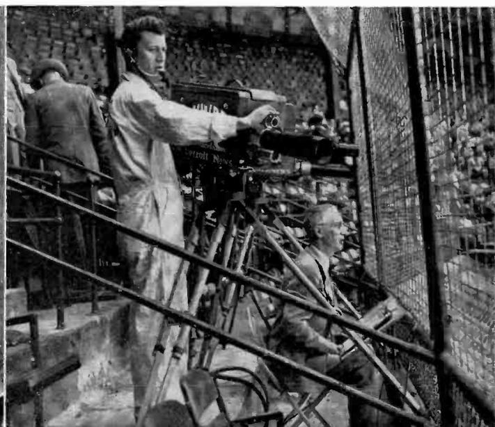
WVDT, Detroit (Tigers) uses two RCA TK-30A Cameras. Both are at the same location, in the lower stands just behind homeplate. Since the pictures above were made, shatter-proof glass has been substituted for the section of the screen which the cameras shoot through. Using two cameras, the 90MM and 135MM lenses are used for general coverage, with the 15" and 17" lens used for closeups.
