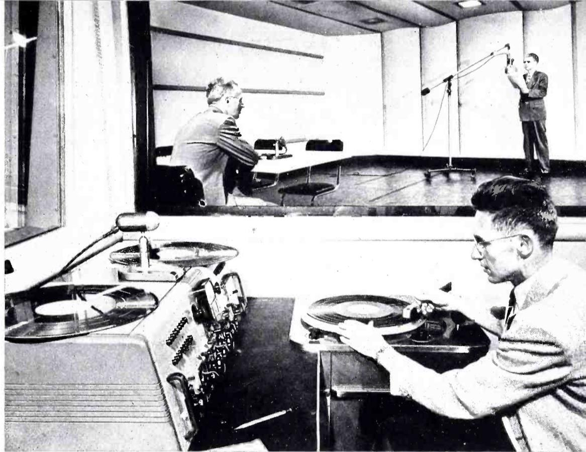
**FIG. 9.** (At Right) Looking into studio "B" from the main control room which is designed to control both studios. Equipment consists of an RCA 76-B4 consolette, two 70-C turntables and RCA microphones. Large double plate glass windows are used to provide good visibility into studios.
