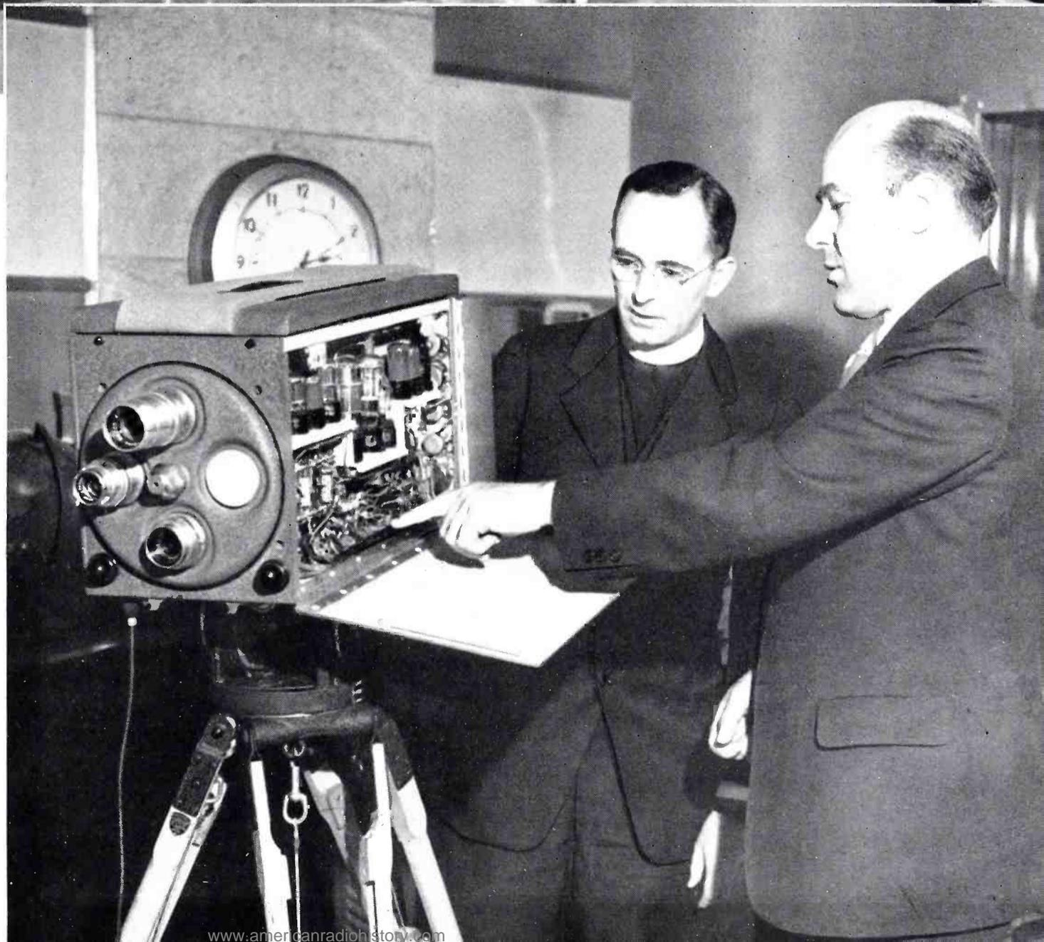
**FIG. 3.** (right) An important part of WOW's television program is a contract with Creighton University of Omaha for cooperation and collaboration on television training. In this picture Jos. Herald, Technical Supervisor, is explaining RCA TK-30A to Father R. S. Williams, S.J., Coordinator of Television for Creighton University.
