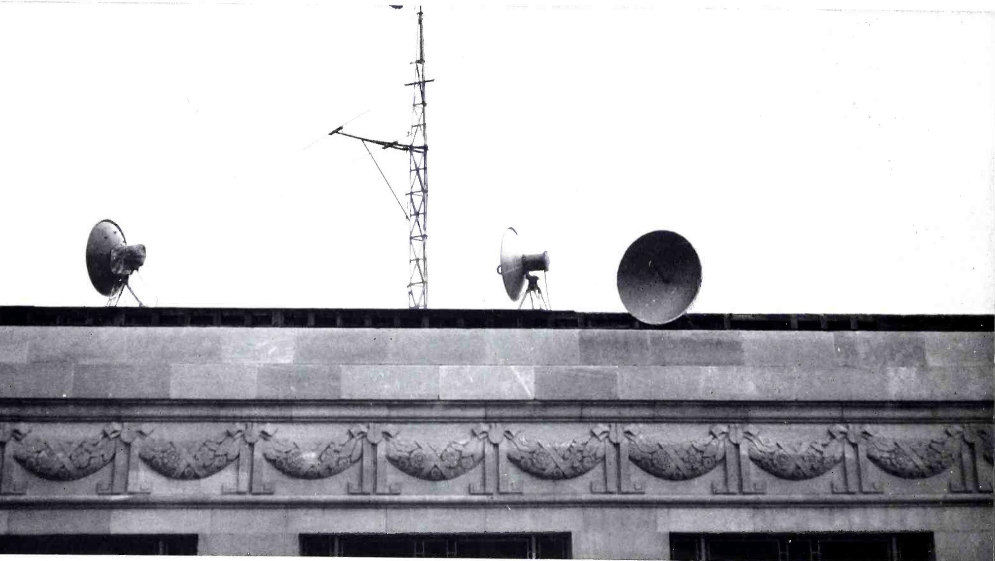
**MICROWAVE RELAYS.** most of them using standard RCA equipment units, were employed between the various pickup points in Philadelphia. Parabolas on the roof of Convention Hall are shown here. The two on the left are, NBC and ABC receiver units on line from the hotel. Parabola on right is NBC transmitter unit directed to relay system terminal at Wyndmoor. Structure on tower is old low-frequency antenna.
