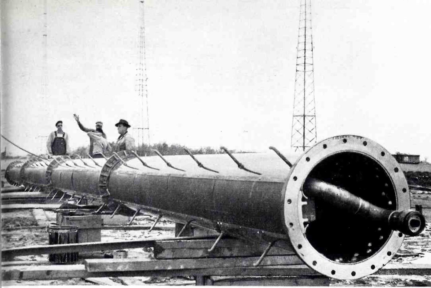
FIG. 11 (above). Here is the top unit—all four standard aluminum sections bolted together and complete with transmission line installed and tested.
