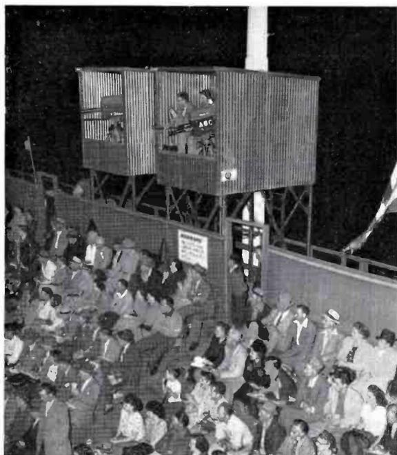
KGO-TV's No. 2 and No. 3 Cameras are mounted in these specially-built booths along 1st base line. No. 2 covers infield play, No. 3 (using Zoomar lens daytimes) the outfield play.
