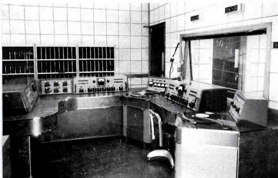
faces the studio control room window. From this position, the operator has access to both consolettes, both turntables—and as previously mentioned has full view into the transmitter room. Note in Fig. 2, how a special turret was installed between the consolettes. This serves to accommodate essential remote meters, tower indicating lights and city or auxiliary power indicators.
