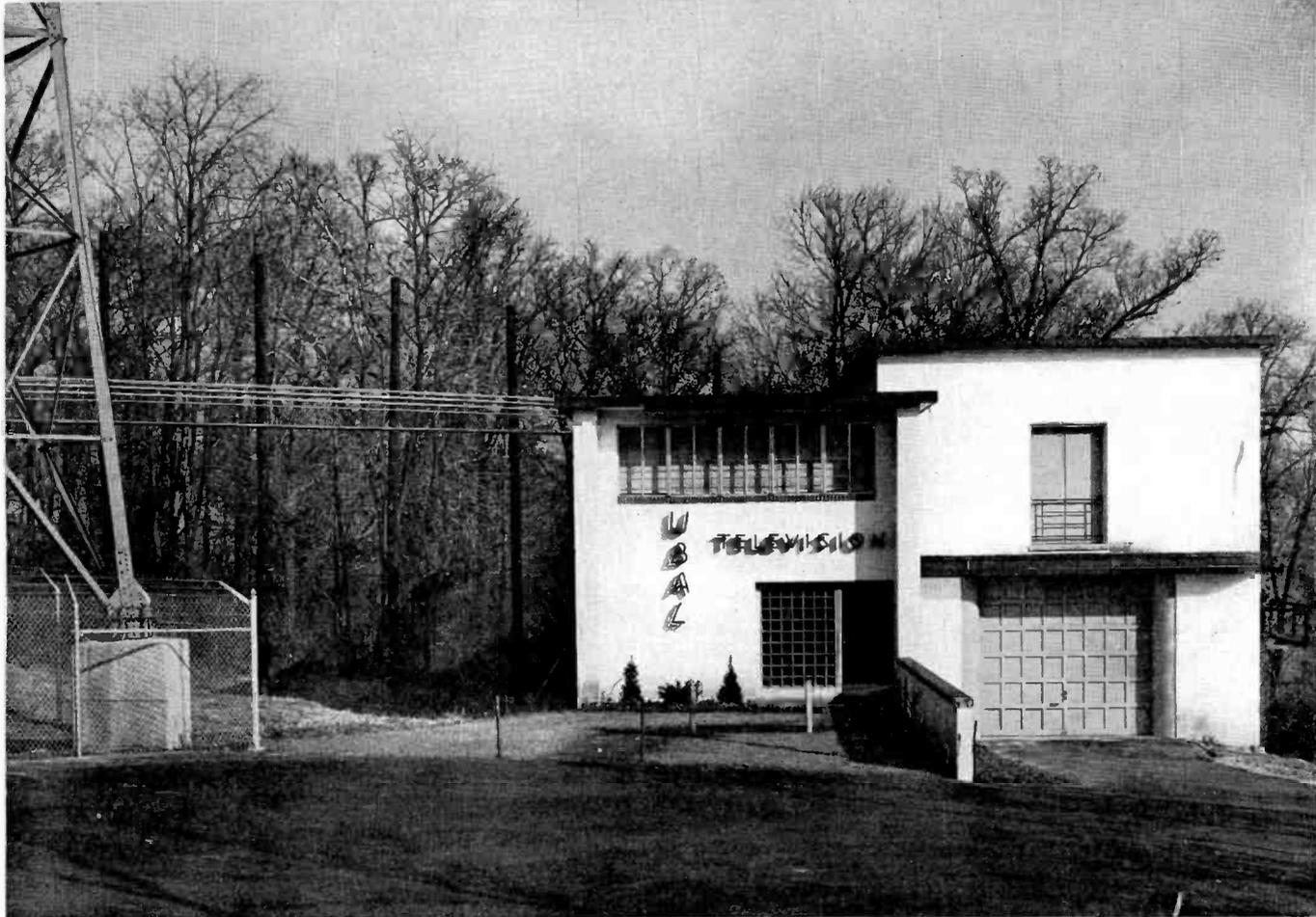
FIG. 12. The modern transmitter building contains a garage for Mobile Unit, workshop, office, kitchen, and the transmitter room. Feed lines, supported by several sturdy poles, are routed up the tower (left) to the 6-section Superturstile.
