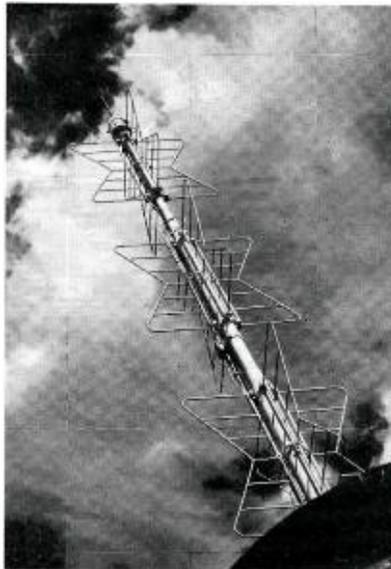
FIG. 1. Closeup of XHTV's Super Turnstile Antenna which tops Mexico City's skyline.
