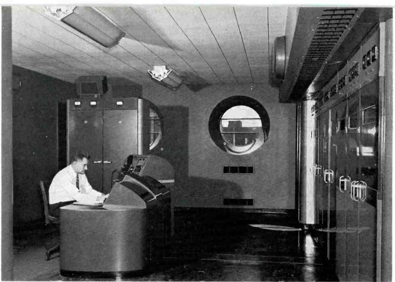
FIG. 6 (above). Transmitter Room view showing flush mounted RCA transmitter, Supervisory Control Console and equipment racks. Mr. Gordon Rustemeyer, Transmitter Supervisor, is shown at the controls.
