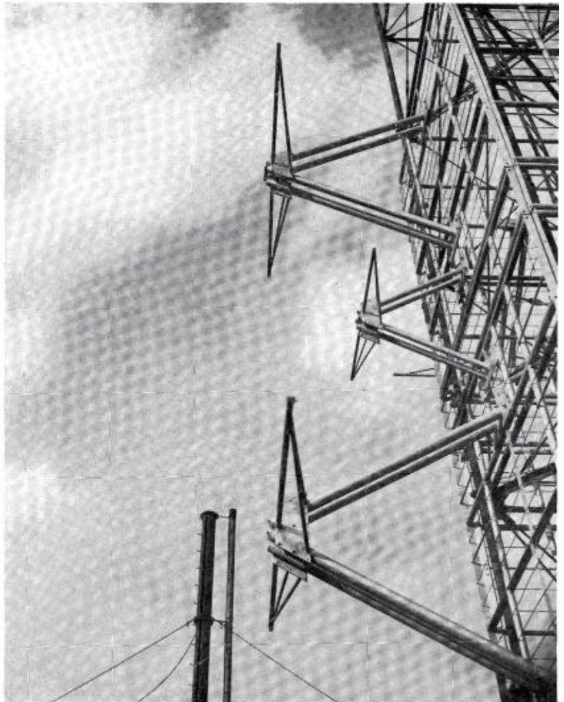
FIG. 14. FM Dipole Located in the Channel 2 Array.
