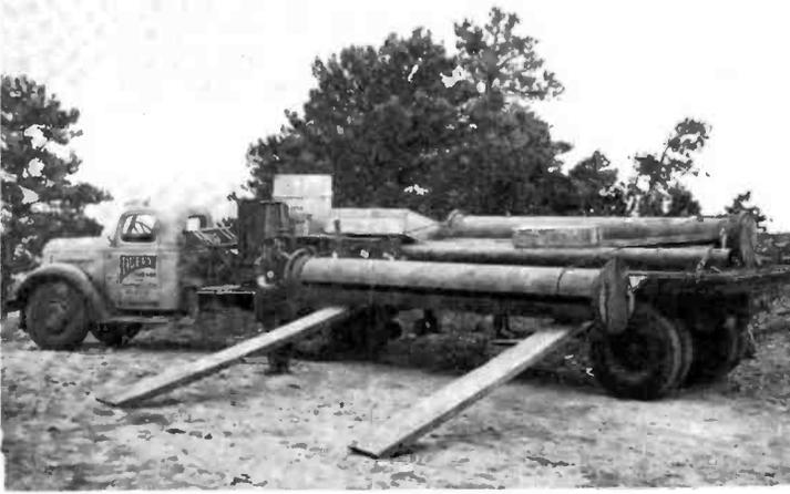
FIG. 9. Part of the two-section FM Pylon being unloaded at the site.
