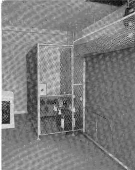
FIG. 6. Rear of transmitter enclosure showing metal guard for high-voltage bus, and inter-lock fence for plate and modulation transformers. Spun glass filters provide air intake through external louvres. Door to this room not interlocked, permits inspection during operation.
