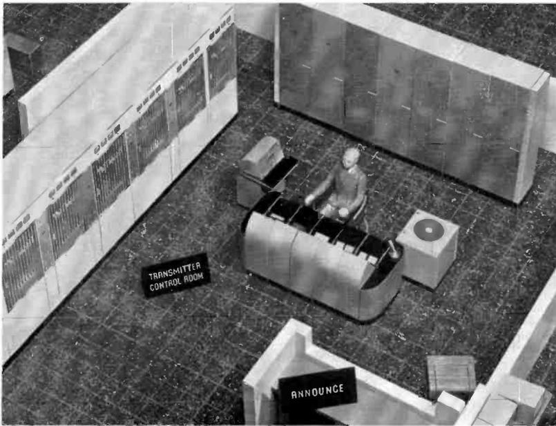
FIG. 36. Model layout illustrating how the TS-1A Master Switching Panel can be housed in the RCA, MI-14905 table turret combination and conveniently located near the operating consoles.
