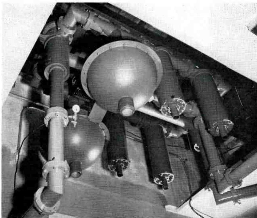
FIG. 2. The RCA Filterplexer (combination sideband filter and constant-impedance notch diplexer) is shown inverted and suspended from ceiling. See Fig. 4.
