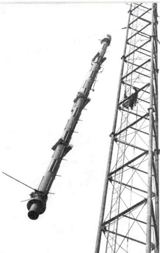
FIG. 3. Checking progress every step of the way, tower climbers keep pace with the rising RCA UHF Pylon antenna. This photo was taken as the antenna reached the 300-foot mark.
