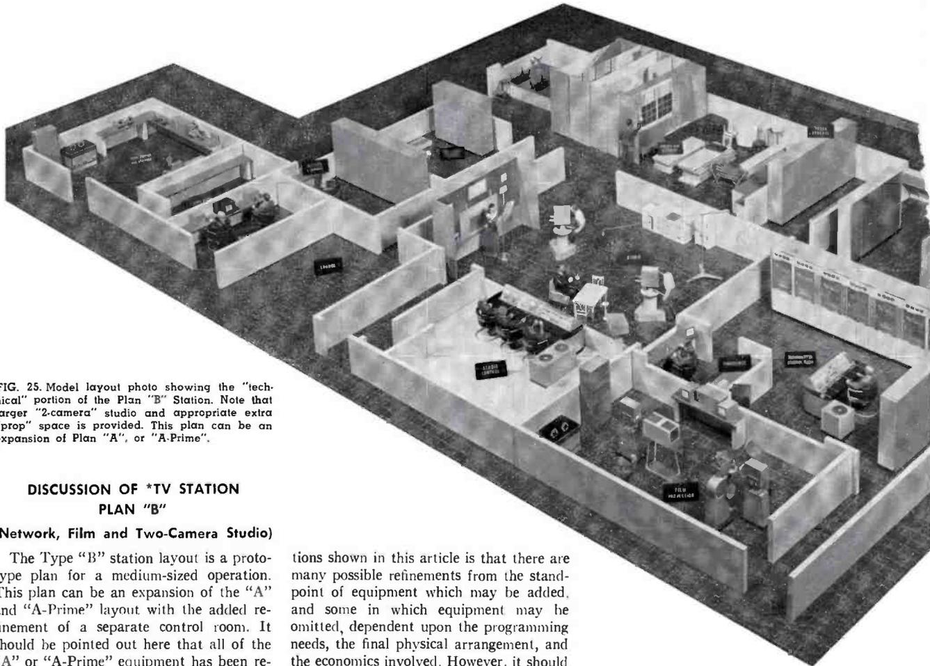
FIG. 25. Model layout photo showing the "technical" portion of the Plan "B" Station. Note that larger "2-camera" studio and appropriate extra "prop" space is provided. This plan can be an expansion of Plan "A", or "A-Prime".
