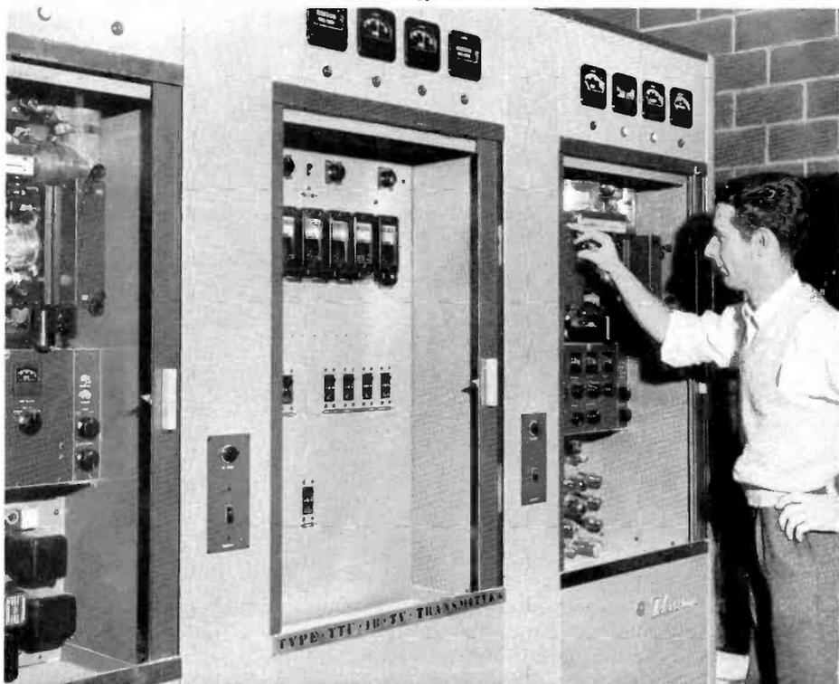
transmitter, the transmitter was operated without the dust filters. Clouds of dust have settled in every portion of the transmitter to be possible sources of outage. Two hours of air time were lost when this dust provided a firing path for the final amplifier plate voltage around one of the insulating micas in the tuned cavity. Simple precautions against dust would have prevented this occurrence.
