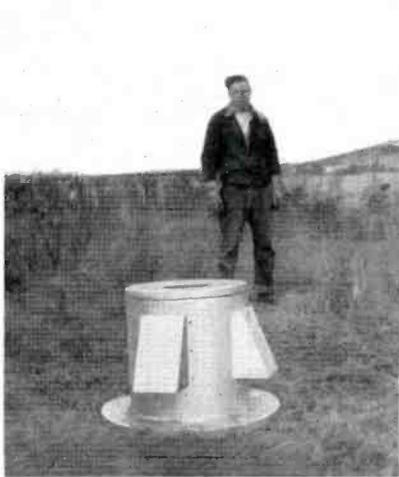
Fig. 9. View of Flange Pedestal Adapter used to mount the UHF Pylon antenna atop the FM Pylon. Wedge-shaped extensions are vent louvers.
