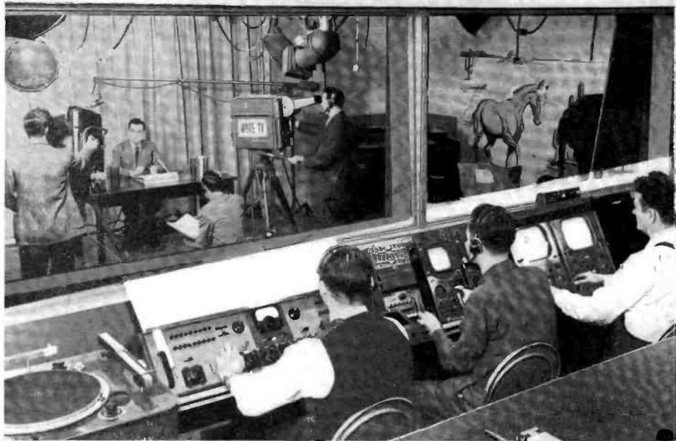
FIG. 4 (center). Control room at studio houses field camera monitors, film and program monitors, off-the-air monitor, and racks for sync generator, monoscope, and allied equipment. High desk in rear will be switching position to be used by program director in controlling cameras and film on studio-produced shows.
