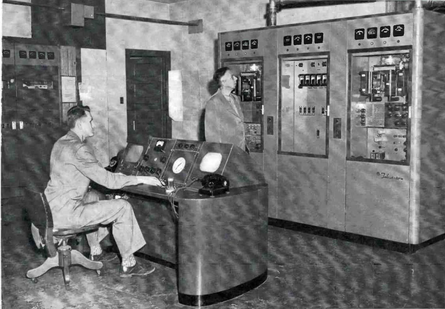
FIG. 2. Main room of TV transmitter building. Charles Sakoski, Sr., Chief Engineer, checks 1 KW RCA UHF transmitter, while Joe Emashowski, Jr. operates console. In the rear is 1 KW RCA FM transmitter. Room through door in rear is workshop and store-room.
