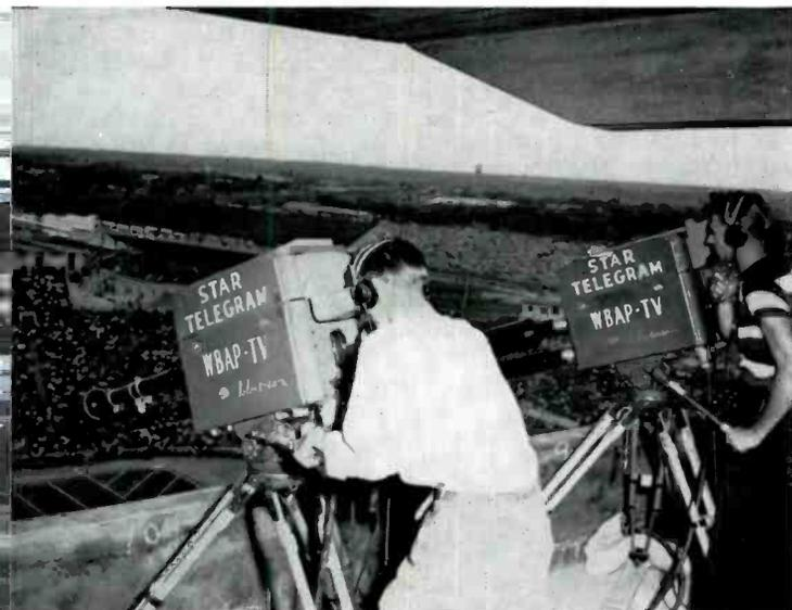
FIG. 26 (below). To improve their baseball pickup (cameras in press box were too high) WBAP engineers rigged up this "cowboy camera" in the Ft. Worth ball park.
