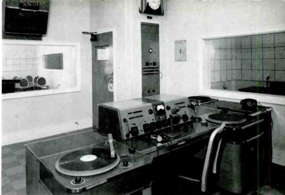
FIG. 15 (center). This view of the latest large studio shows the junction of the polycylindrical diffusers with a blanket wall under Transite. A part of the serrated ceiling is also visible. The control room at the right has a full view of the entire studio.
