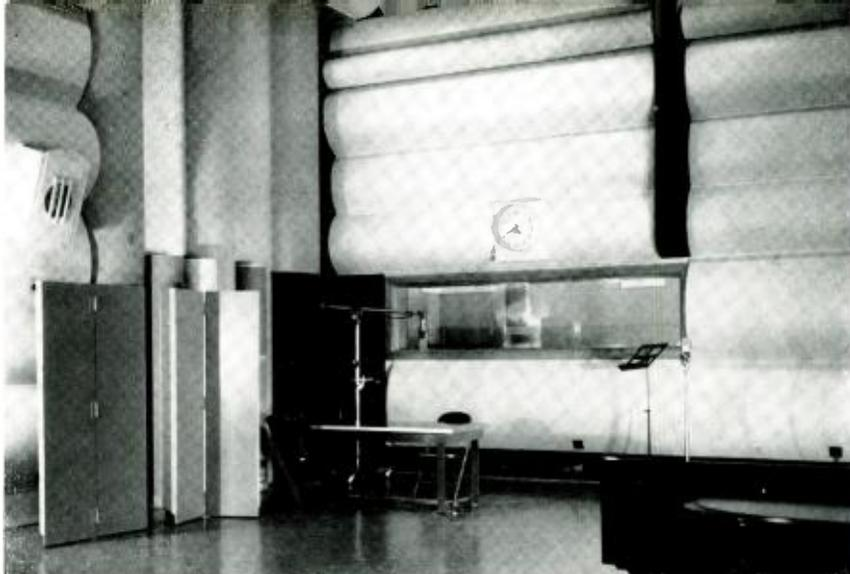
FIG. 28 (right). A corner of Studio B, which is identical to Studio A, thereby giving added flexibility for rehearsal and programming. Each studio has an "announcer's delight" control box (far corner) from which position he can do his own switching when he makes announcements. Note the cowbell (WBAP's identification for thirty years) at each announce position.
