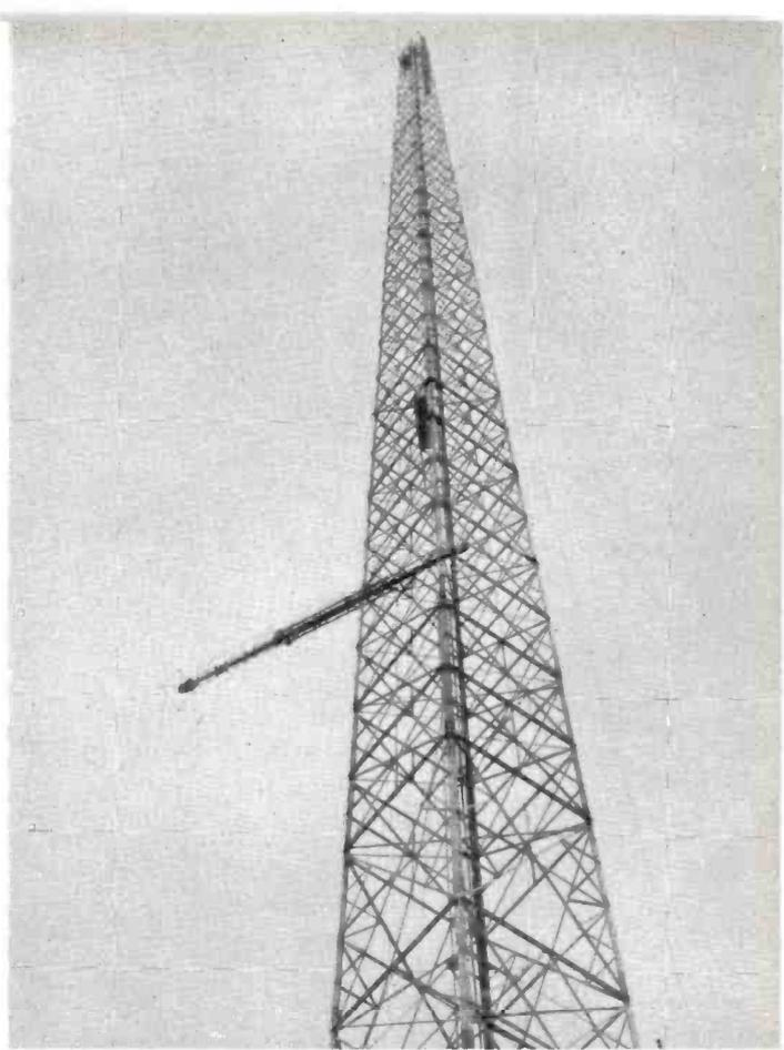
FIG. 13. The 6-bay RCA Superturnstile antenna half way up. The antenna was placed on top of a 441-foot Lehigh tower making the overall height of 480 feet.
