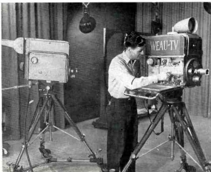
FIG. 11. A corner of WEAU's studio is devoted to daily weather reporting. The Weather Man stands behind the glass map and letters the map with weather reports, however, they appear reversed on the camera side of the map. A reversing switch was placed in the horizontal sweep of the TK-11A camera to again reverse the map. The reversing idea belongs to Mr. Richard Kepler, TV Manager for WEAU.
