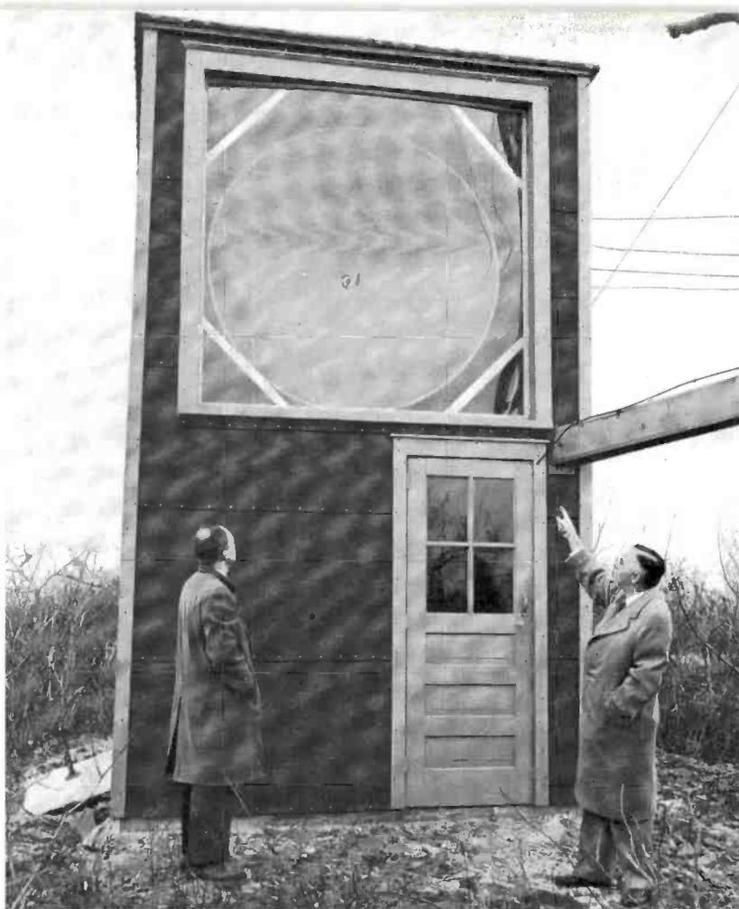
Closeup of relay transmitter housing at Pimple Hill. Network service is relayed from this point. 70 miles air distance from New York. Pimple Hill station is the main inter-city relay connection. ▲
