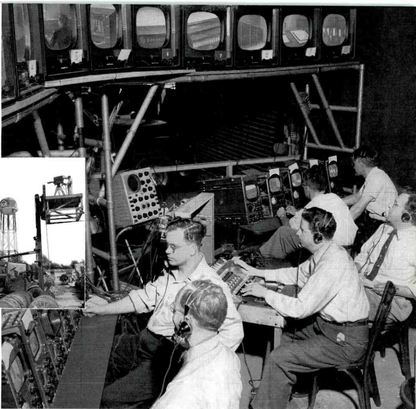
FIG. 9. Magnitude of Moorestown closed-circuit plant tour is graphically caught by camera during the show. Experienced demonstrations group in improvised studio kept close watch on entire ten camera chains and expertly cut-in sequences at command of program director.
