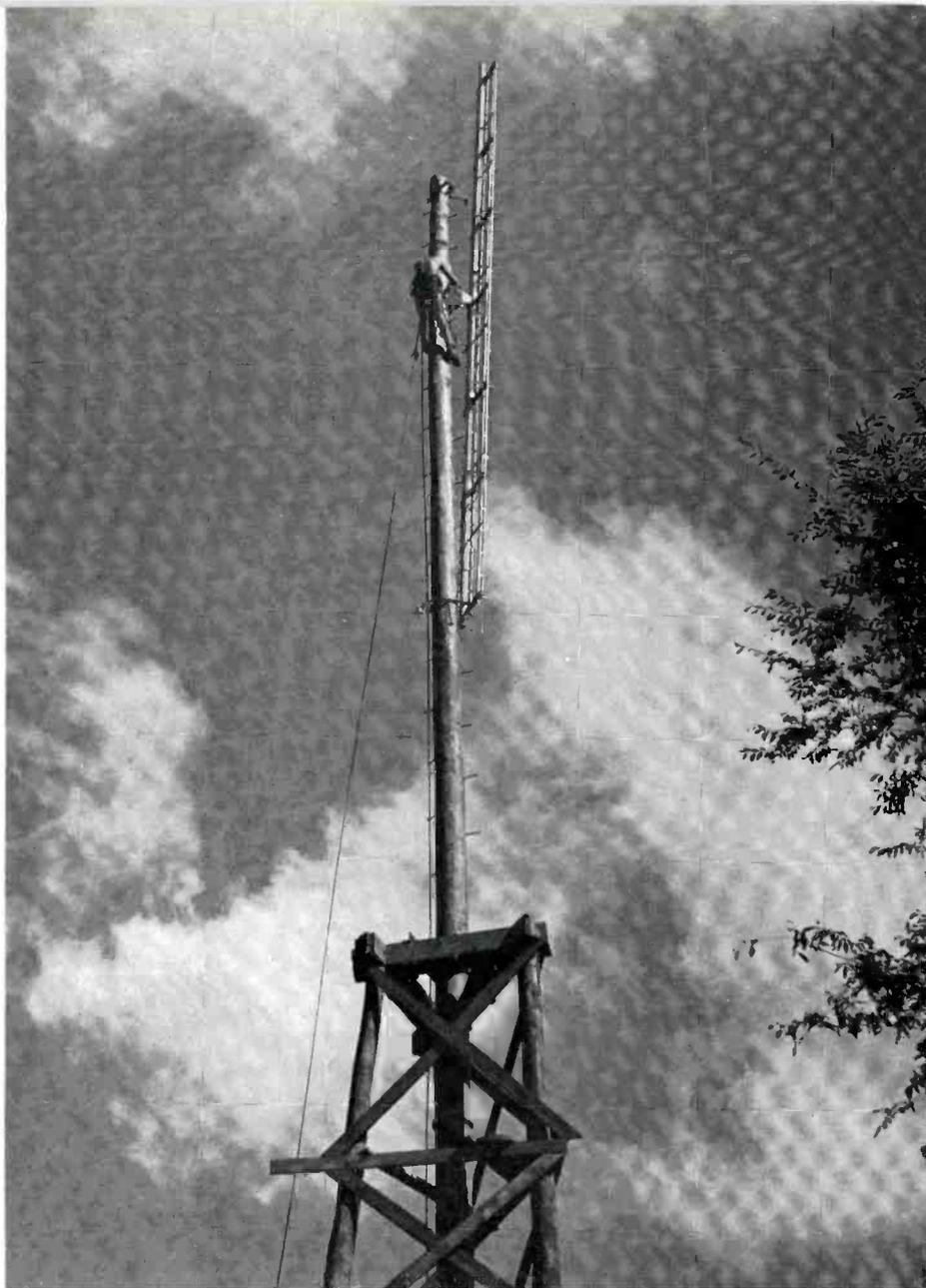
gain, 105 db of attenuation was required. 90 db of this was obtained by separating the antennas 100 feet. The additional 15 db of attenuation was obtained by a feed-back loop connected between the input and output terminals of the amplifier.
