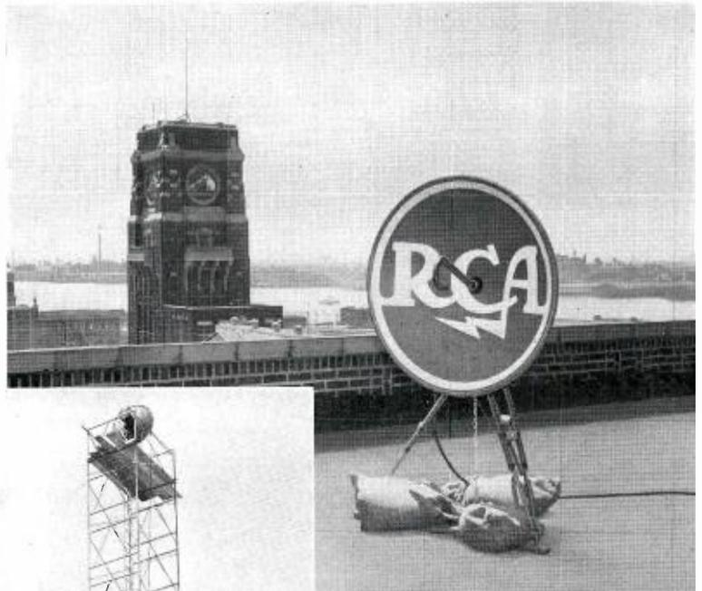
FIG. 8. Microwave installation used for closed-circuit TV tour of Moorestown Plant staged for nation's ranking air chiefs. Above, 4-foot parabolic antenna is moored to roof of RCA's general office building in Camden; below, temporary 70-foot tower on Moorestown Plant from which signals were relayed.
