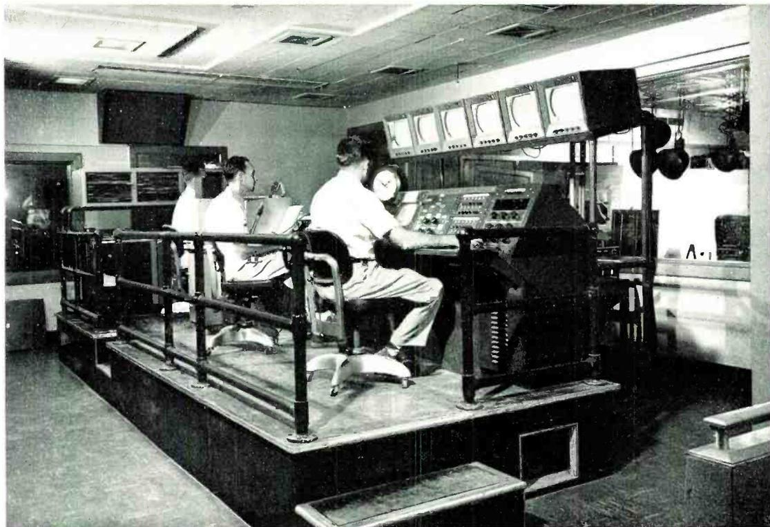
FIG. 12. WBAP-TV's Television Master Control Room (see floor plan Fig. 8). Audio engineer, program director and technical director sit on raised platform. The six monochrome camera monitors are mounted above the studio window. The three color camera monitors are located just below these and are not visible in this view.
