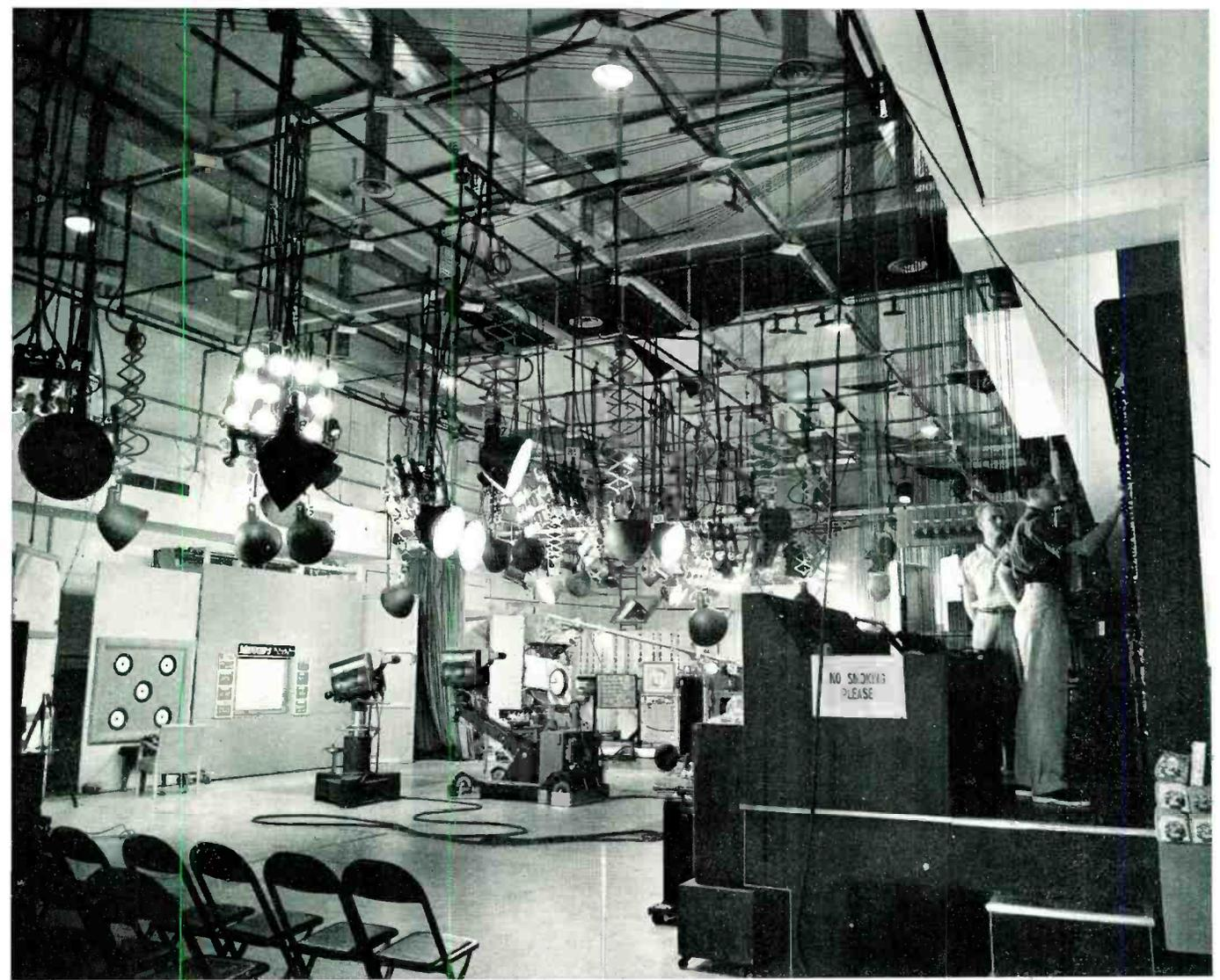
FIG. 19 (above). This view of WBAP-TV's Studio 1 gives a good idea of the lighting as rearranged for color. Main light complement consists of thirty scoops, mounted on pantographs, 20 TV Associates Fixtures, and thirty spots mounted on catwalk around sides of studio. Lighting is controlled from a new light bridge (right in above view) which is on the studio floor for easy access.
