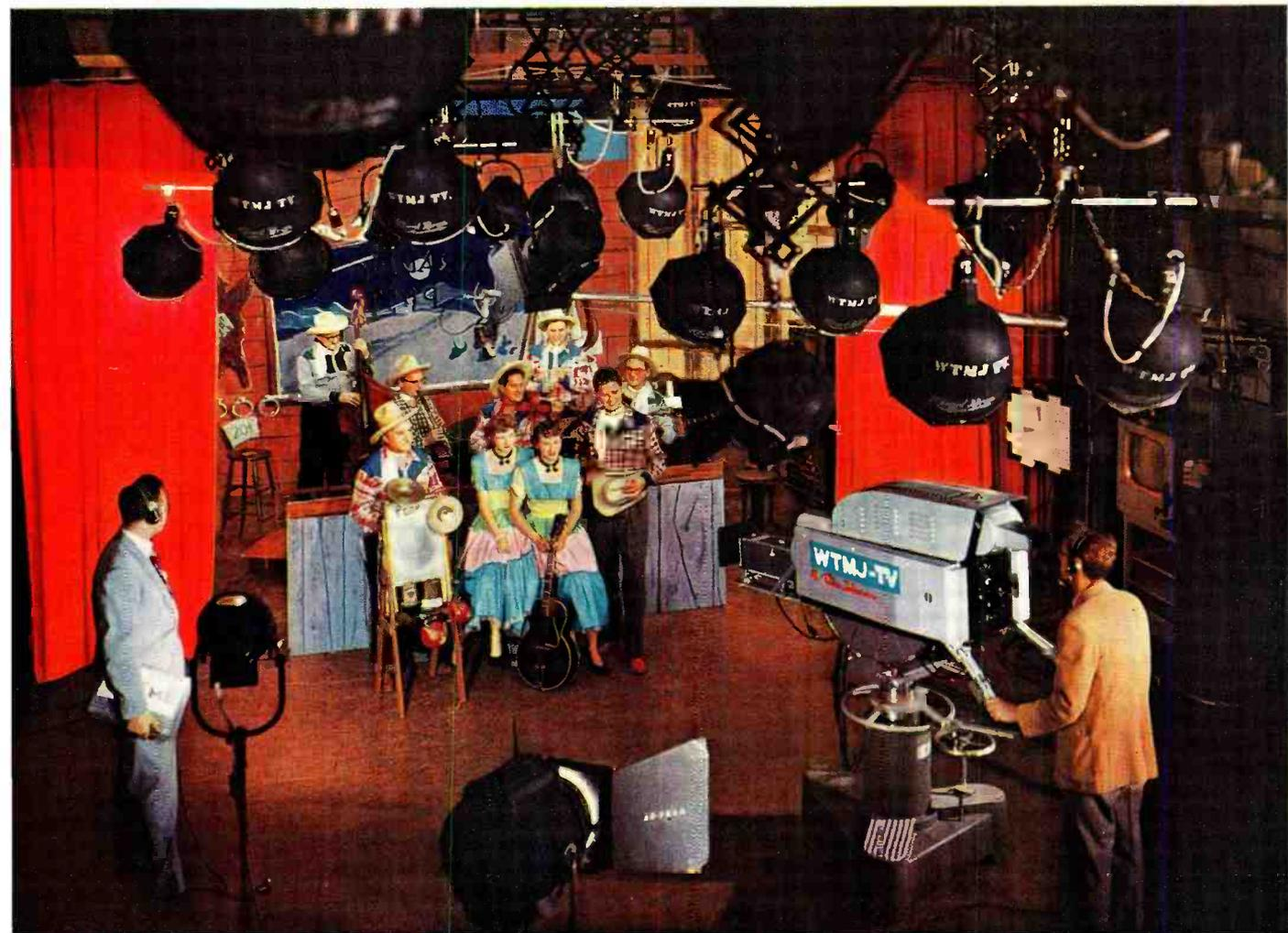
FIG. 13. This is the "Trading Post" set used on WTMJ-TV's color telecast of "The Hotshots" program. Standing in front of the board fence are "Pedro" (Alex Mayer) and Gordon Hinkley, m.c. of the Hotshots, and the Winkert sisters. Note the Electrazoom lens which gives WTMJ-TV almost as much flexibility as a second camera, and saves the labor of "dollying" in and out.
