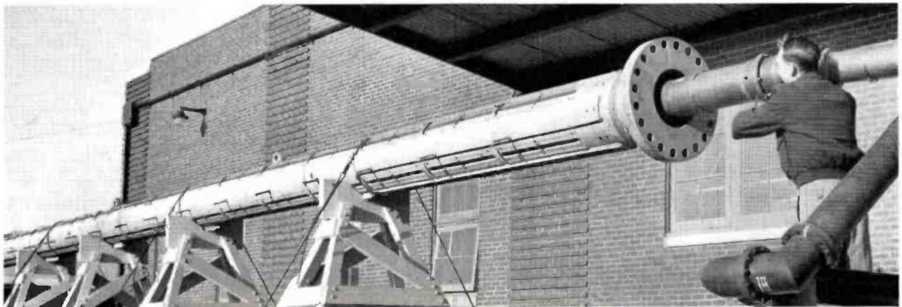
Approximately 4½ megawatts are produced by feeding 100 kilowatts into this super-power antenna with a gain of nearly 50.
