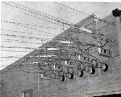
FIG. 6. Building dead-end termination of open wire line leading to five towers. Lightning protector horn-gaps are visible above each ground plate.
