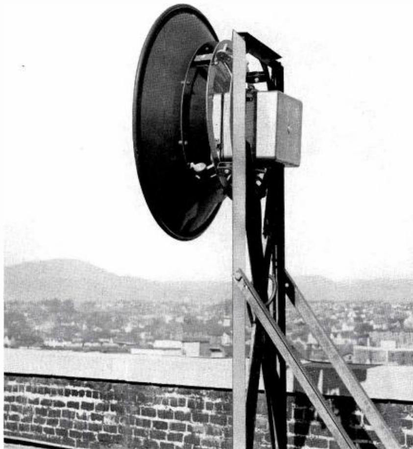
FIG. 7. Side view of microwave installation at Roanoke terminal showing 4 foot parabolic reflector with head end transmitting equipment and angle iron supporting frame.
