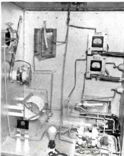
FIG. 13. Line terminating unit interior showing switch for day/night patterns. Two meters are for day current and night current measurement.
