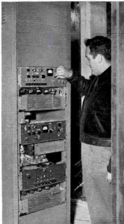
FIG. 13. Engineer Oliver Lienhard adjusting microwave equipment in relay station building at Poor Mountain.
