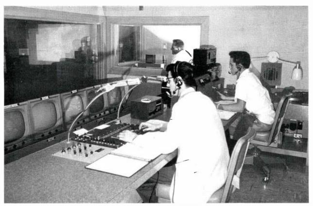
FIG. 13. View of studio "B" production control with announcer's booth in the background. Desk equipment in this control room is similar to that of control room "A", permitting familiarity when operators and directors switch from one room to the other.
