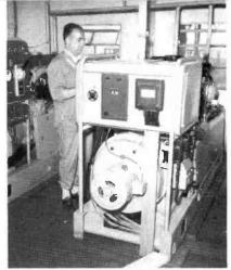
FIG. 21. Two emergency power units of 93 kw and 600 kw are available to power TV and radio equipment at M. Penice transmitting site.
