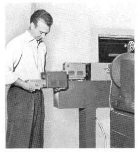
SPARE CAMERA! Simplicity and small size of RCA TK-21 make it practical to keep a third camera on hand as a spare. This allows either film chain to be quickly returned to service in emergencies and provides station clients with this assurance of continuous programming.
