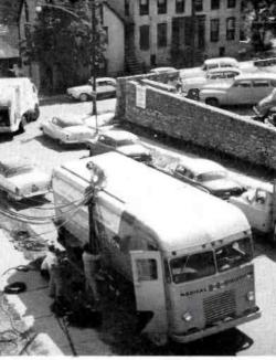
FIG. 13. Mobile unit is parked alongside hospital and connected to studio and power supply via cabling carried in the truck.
