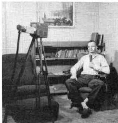
FIG. 9. Live weather casts originate from the engineers' lounge using a TK-21 camera mounted on a tripod.
