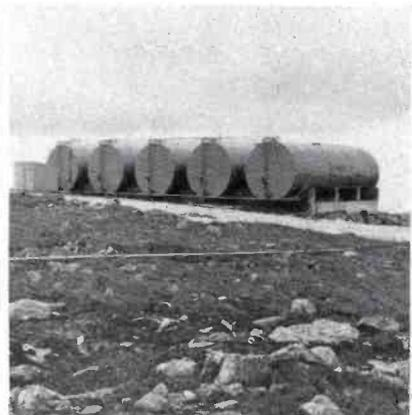
FIG. 10. WMTW's fuel is stored in five 20,000 gallon tanks. These tanks hold a full year's supply of fuel.
