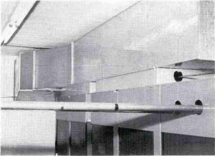
FIG. 9. Duct work on top of transmitter cabinets exhausts hot air to outside of building.
