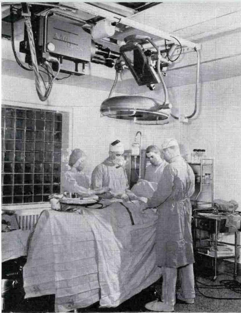
FIG. 9. Medical Color TV Camera is always focused on operating field by means of a mirror used in combination with a special ceiling light, which has a hole in center. Mirror movement and lens switching are remotely operated from the basement control room.
