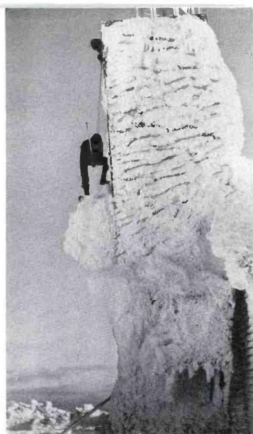
FIG. 4. "Deicing" of antenna tower often requires a pickax and a strong back. Antenna is deiced electrically.
