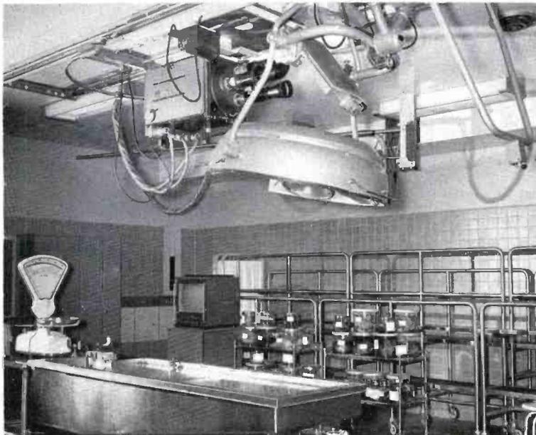
FIG. 11. Ceiling-mounted camera can be swung through full 360 degrees. Travel in north-south and east-west direction controlled by wall switches.
