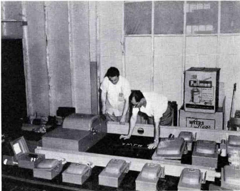
FIG. 12. Power load center is carefully laid out and preassembled. Other units usually assembled on the job, such as water systems and air ducts, were also prefabricated.
