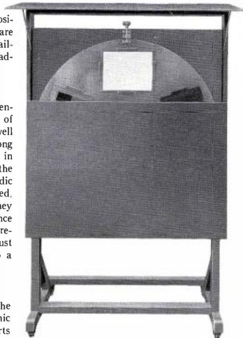
FIG. 5. Front view of television test chart transparency stand developed at NBC.
