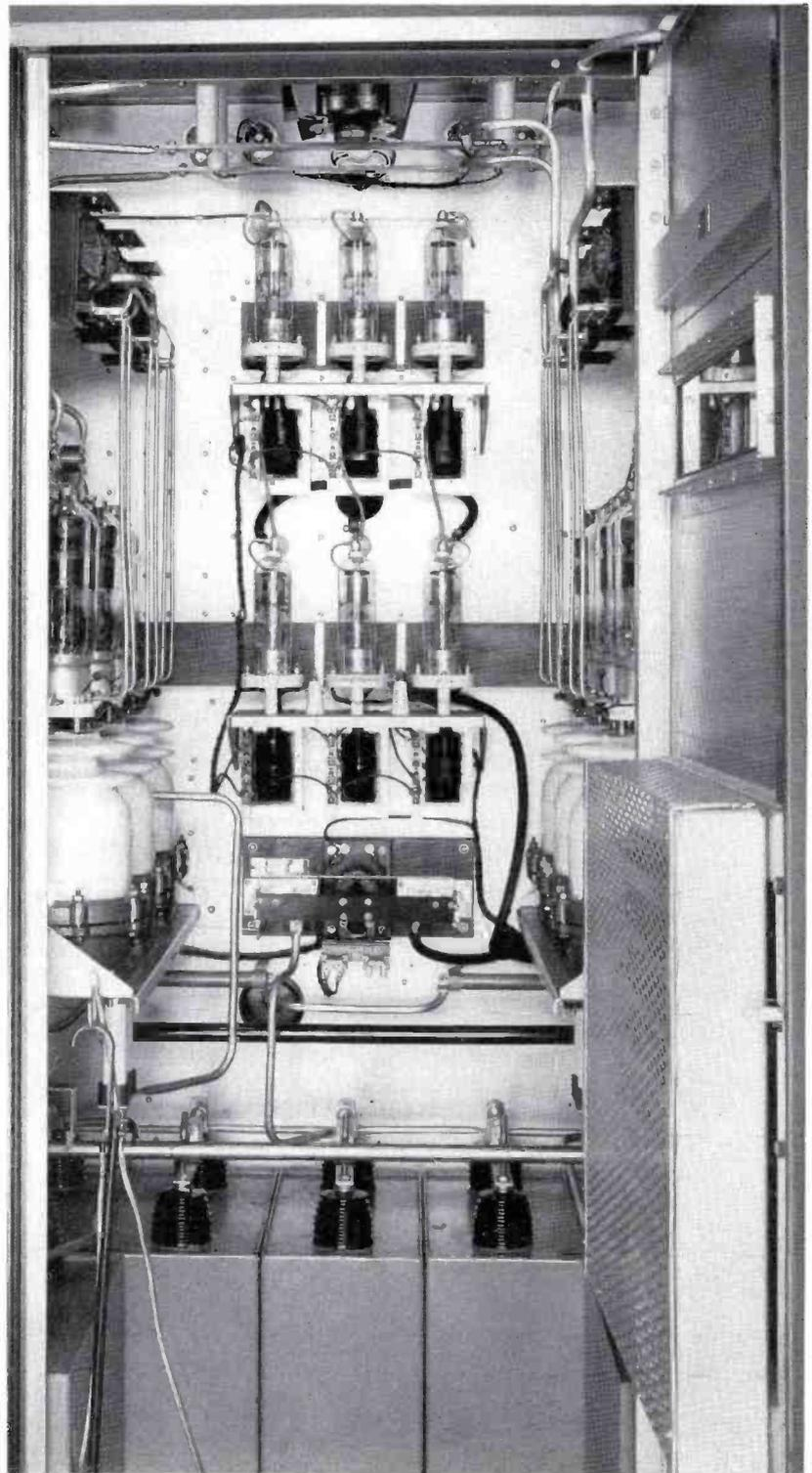
FIG. 13. Front view rectifier and control cubicle.
