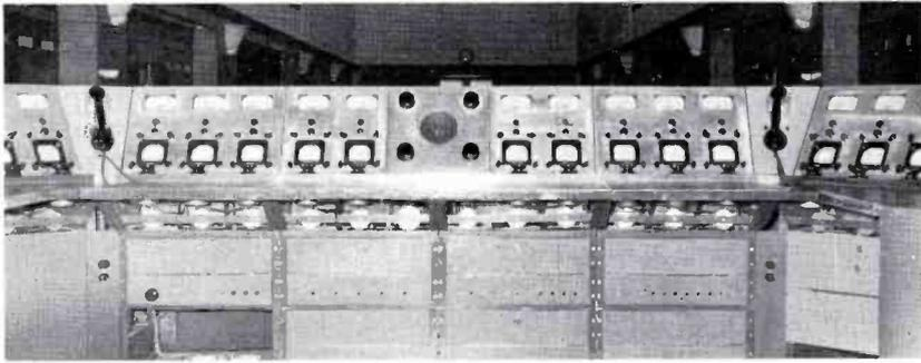
FIG. 41. R-F control console for all transmitters.
