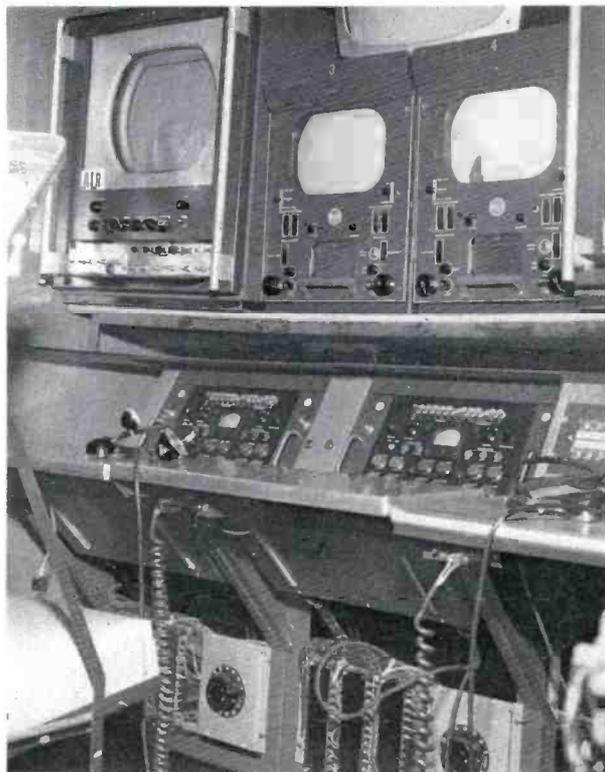
FIG. 20. Camera control positions in remount truck, at left. Switcher position at right. Note equipment is portable and is also used in the studio.
