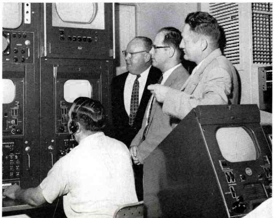
FIG. 7. Inside the mobile unit video operators sit in a recessed area, giving production personnel sitting behind them an unobstructed view of monitors.
