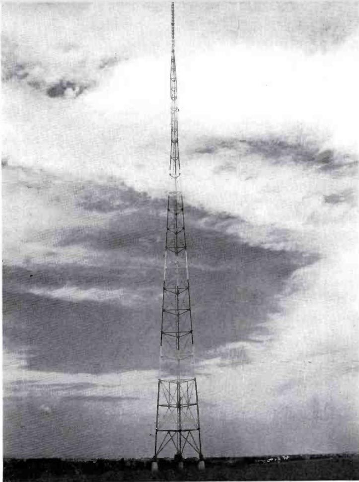
FIG. 14. This is a self-supporting tower. The larger base area supports the entire structure. No guy wires are required.
