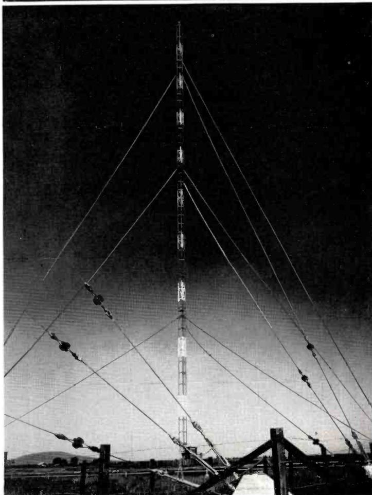
FIG. 15. An insulated-guyed tower and a small building to house the antenna tuning unit is shown here. Observe the insulators used to break the continuity of the guy wires.
