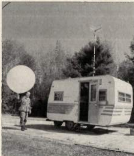
This radiosonde balloon uses a small, battery-powered telemetry transmitter to radio data to the ground station.
