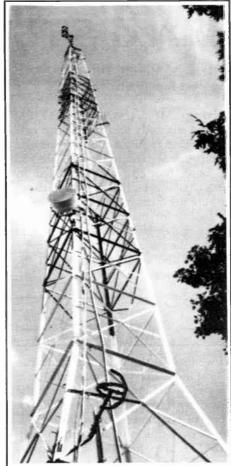
M-A/Com 4' Drum style 21 GHz microwave dish mounted in center of WZZO transmitting
