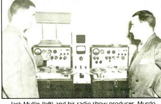
Jack Mullin (left) and his radio show producer, Murdo McKensie looking over Ampex Model 200 audio tape recorder and Magnetophon.
